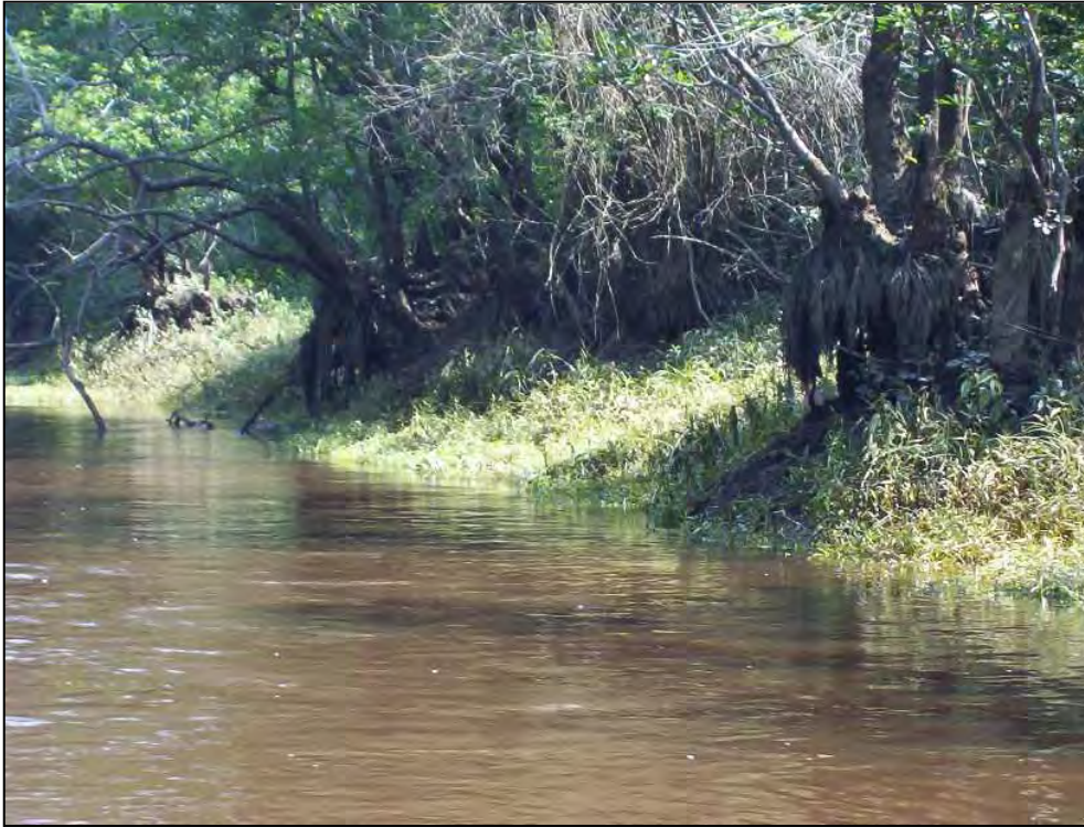
Photo 9. River Observation Point 5. Well established herbaceous vegetation along the banks of the river below the elevation of the former dam crest pool. Little River, Johnston County.
