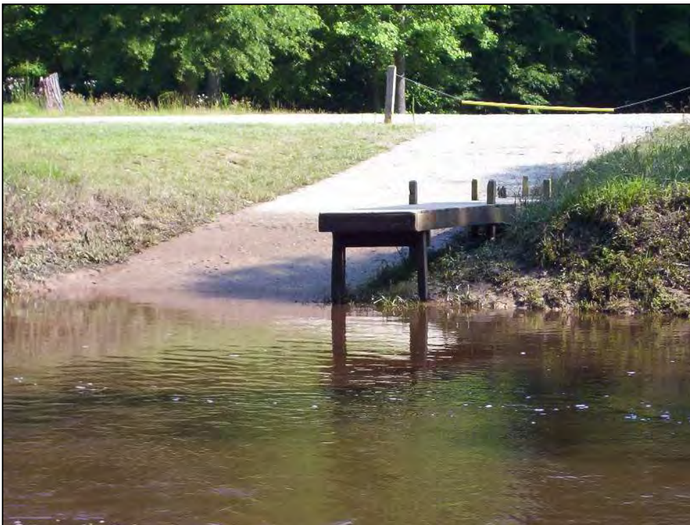
Photo 2. River Observation Point 2. Sediment deposition and high water mark at the Wildlife Resource Commission boat ramp. Little River, Johnston County.
