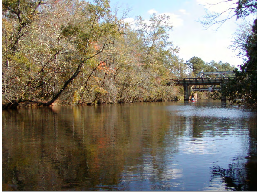
Looking downstream at the US 301 and railroad bridges over the Little River prior to dewatering—note high water surface relative to bankfull elevation
