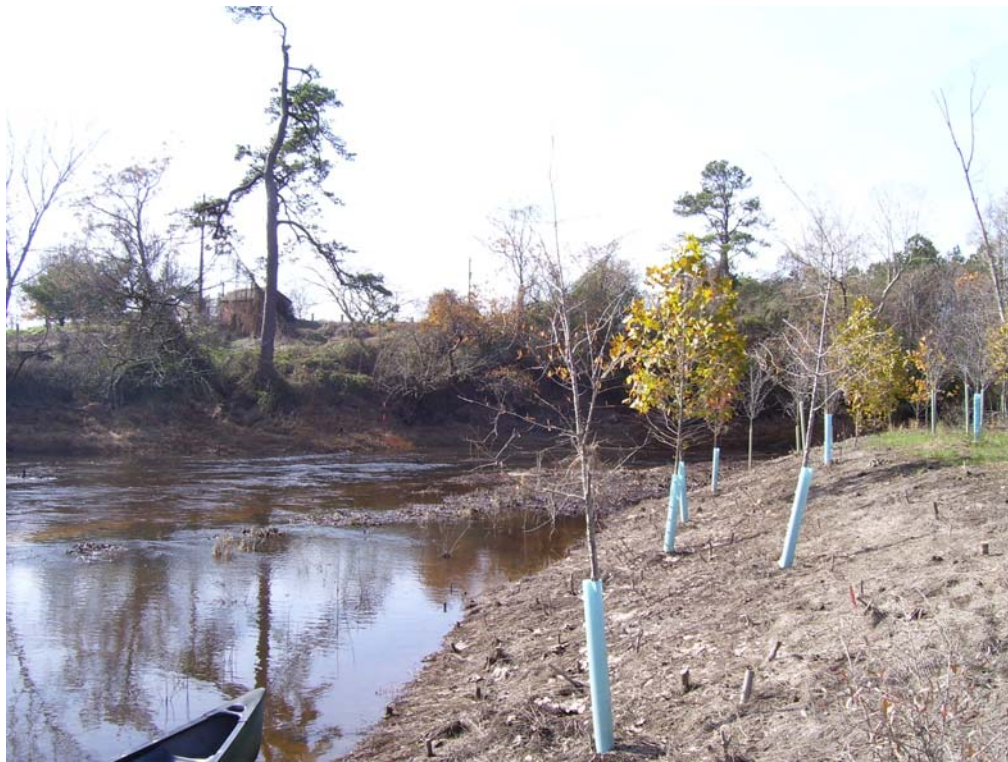
Photo 6. River Observation Point 9. Sediment deposition and elongation of the constructed point bar located at the inside bend of the river at the former dam site. Note the slack water at the over widened reach of river at the toe of the remnant dam structure. Little River, Johnston County.
