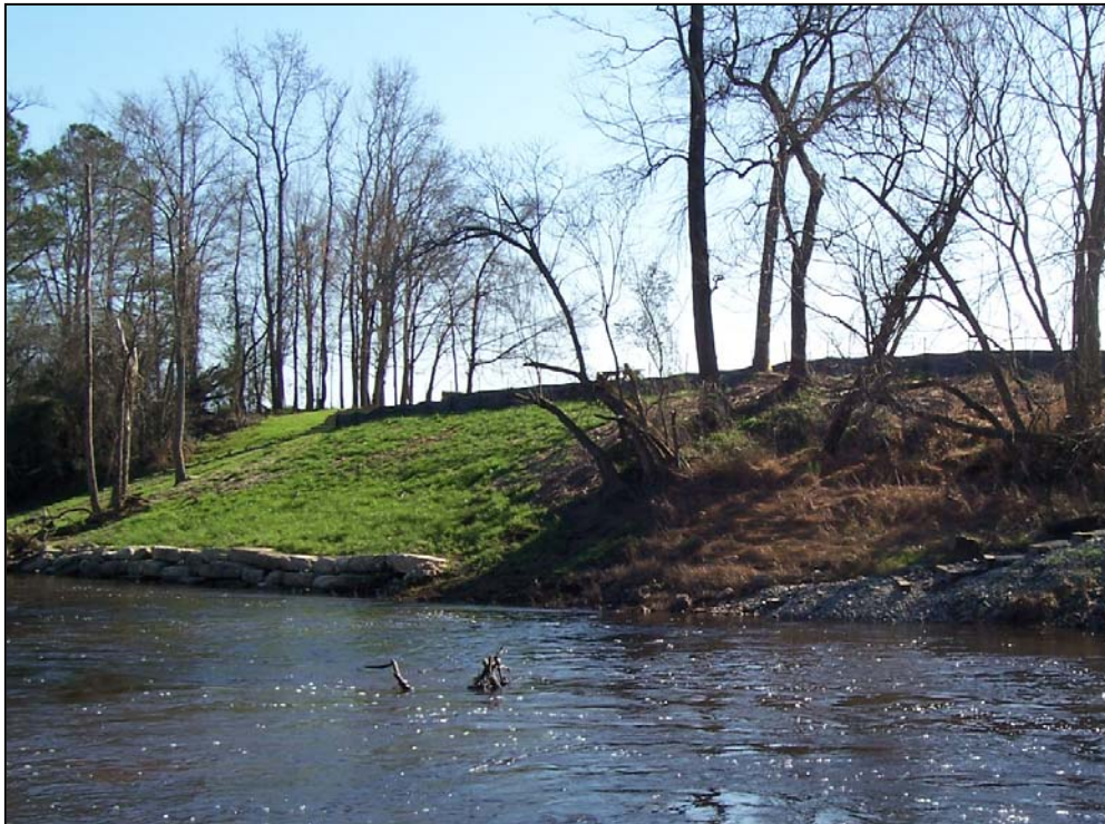
Photo 9. River Observation Point 9: Toe of slope protection and canoe launch staircase along the south embankment. Little River, Johnston County.
