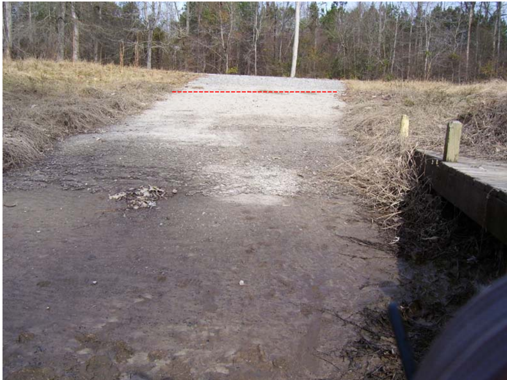
Photo 2. River Observation Point 2. Sediment deposition and high water mark (dashed line) at the Wildlife Resource Commission boat ramp. Little River, Johnston County.
