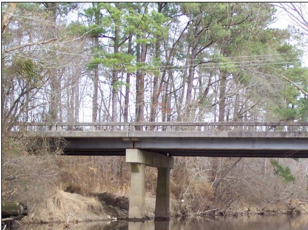
Photo 10. River Observation Point 10: The bridge pilings (Weaver Street) located within the Little River contained no woody debris and no evidence of scouring was observed. Little River, Johnston County.
