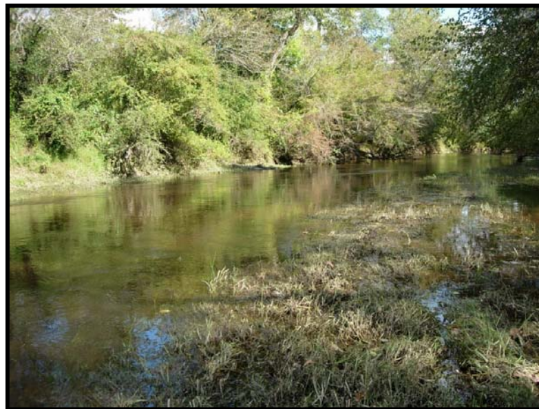
Photo 2. Downstream view of sediment deposits diverting flow away from the right descending bank.
