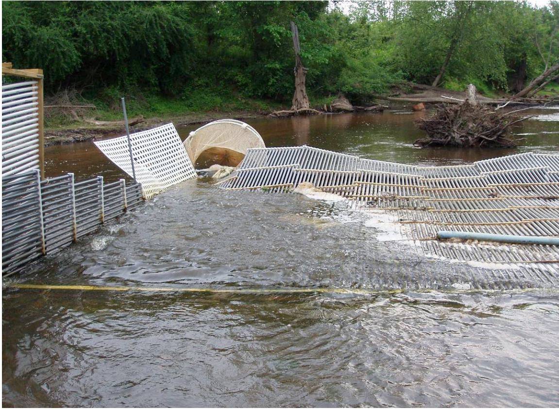
Figure 4. Modification of weir (April 3, 2007) to improve downstream capture of fish. Sandbags sunk portions of the resistance board panels, creating increased flow to the attached net.
