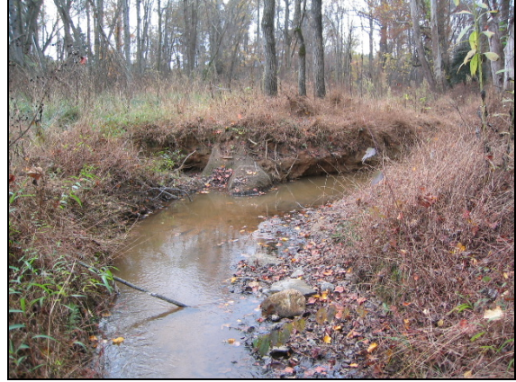
Issue Photo 7 – Station 15+00 Bank Failure under matting.
