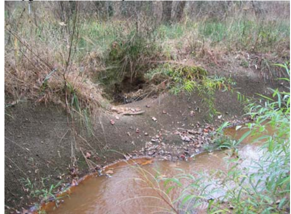
Issue Photo 2 Lyle Creek Pool near station 11+90. Typical Bank Failure on Left Bank
