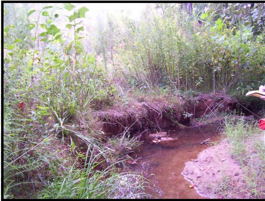
Figure 1— Typical Bank Scour
