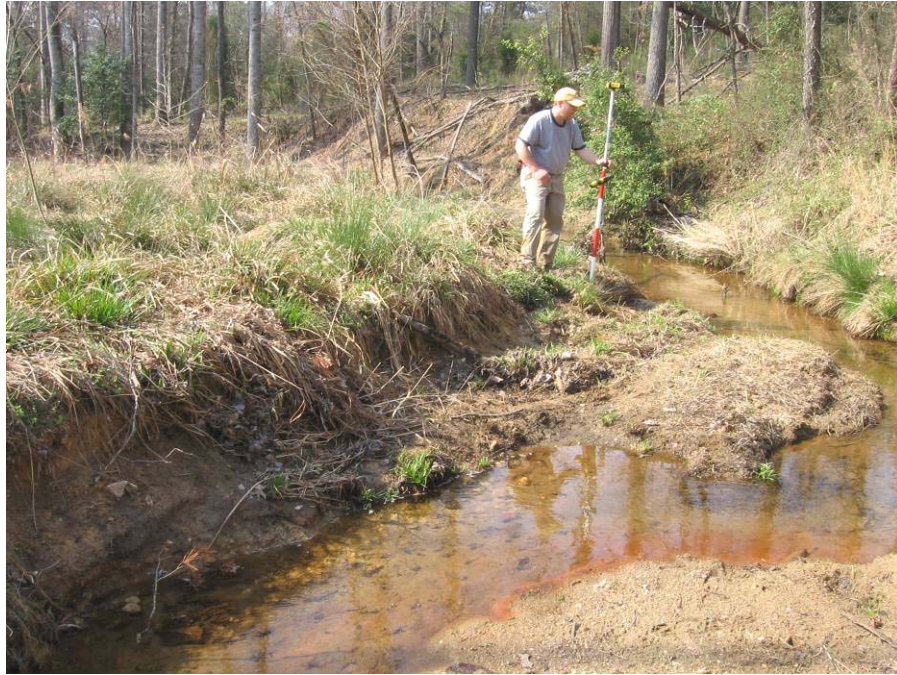
1. Bank Erosion: Moderate-3/30/06
