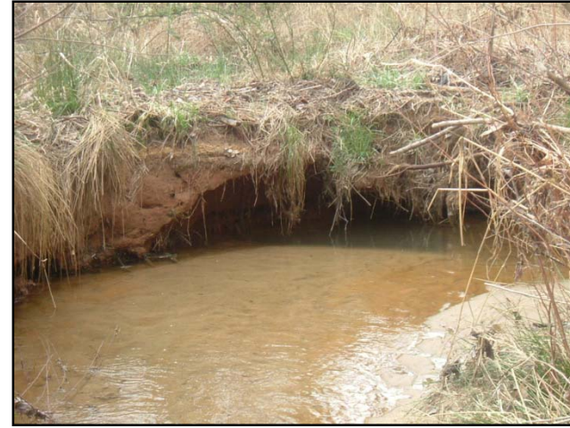
2. Severe Bank Erosion-3/22/2007
