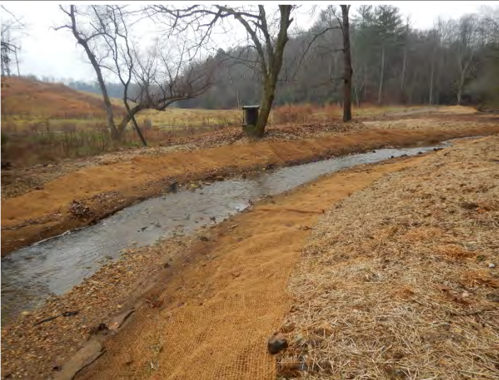
PHOTO POINT 9 Hank's Branch R2 – upstream (01/25/2021)
