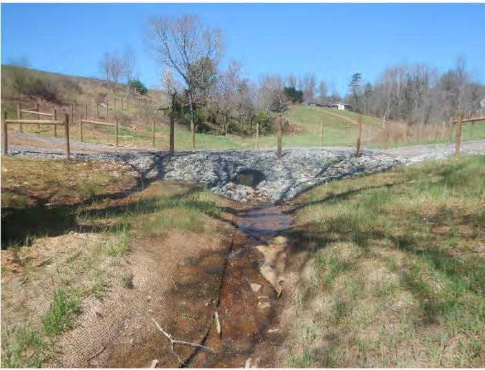
UT1 - Looking Upstream (03/29/2021)
