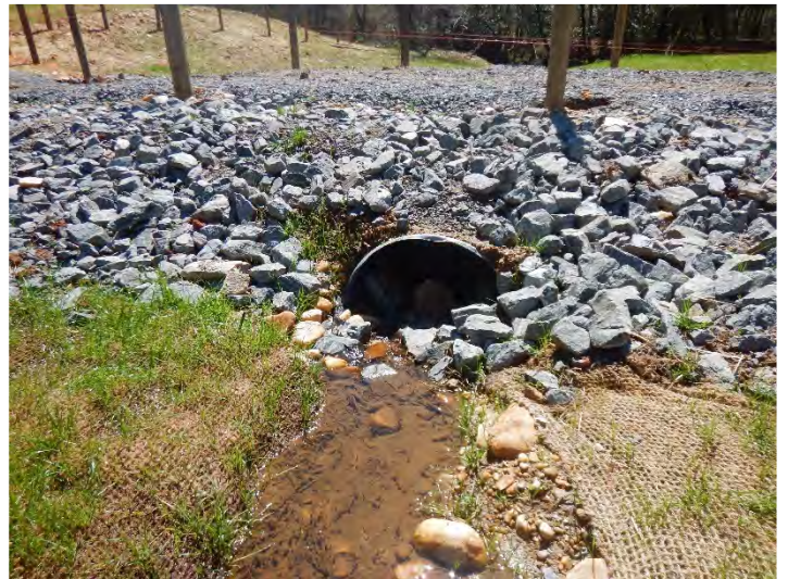
UT5 R2 - Looking Downstream (03/29/2021)
