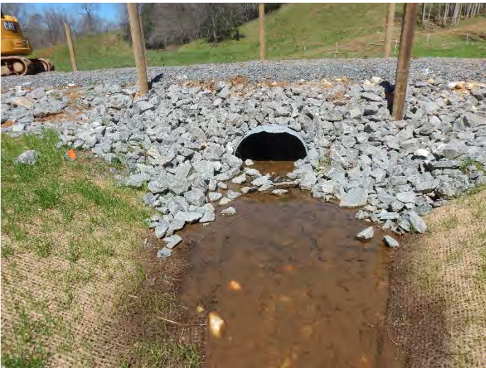
UT5 R2 - Looking Upstream (03/29/2021)
