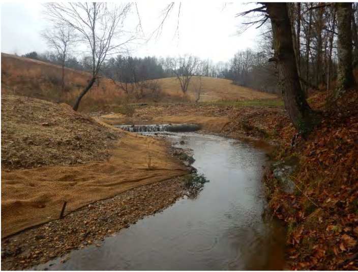
PHOTO POINT 4 Hank's Branch R1 – upstream (01/25/2021)
