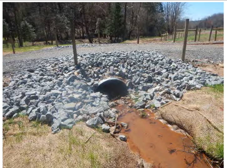
UT3 R3 - Looking Downstream (03/29/2021)
