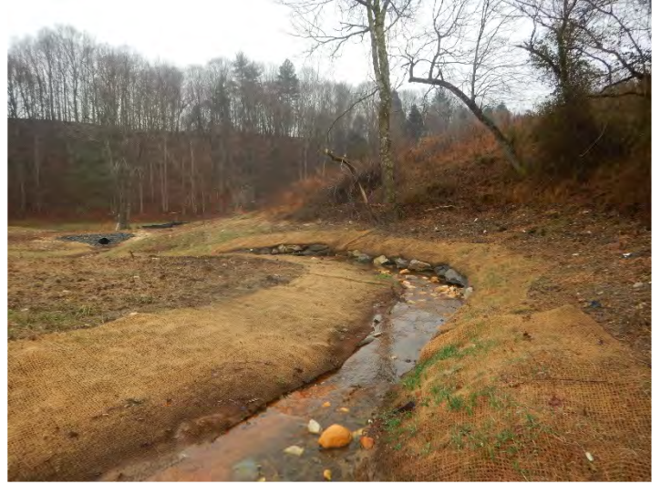
PHOTO POINT 16 UT1 – downstream (01/25/2021)
