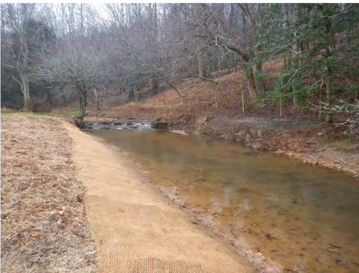
PHOTO POINT 8 Hank's Branch R2 – upstream (01/25/2021)
