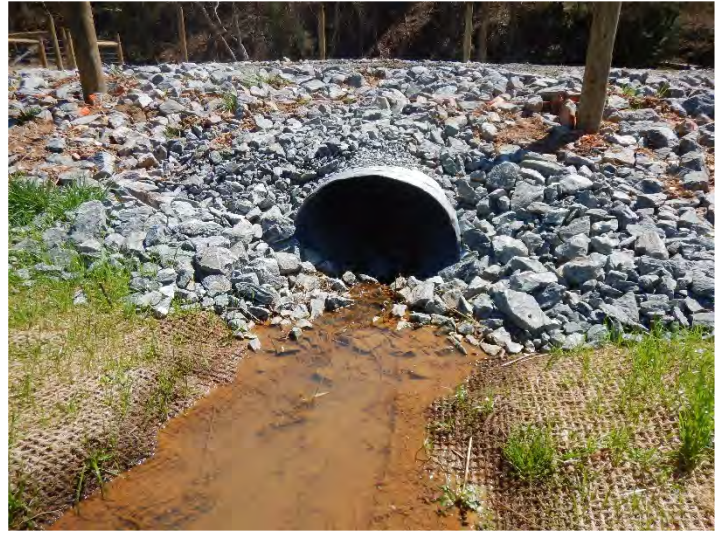
UT4 R3 - Looking Downstream (03/29/2021)
