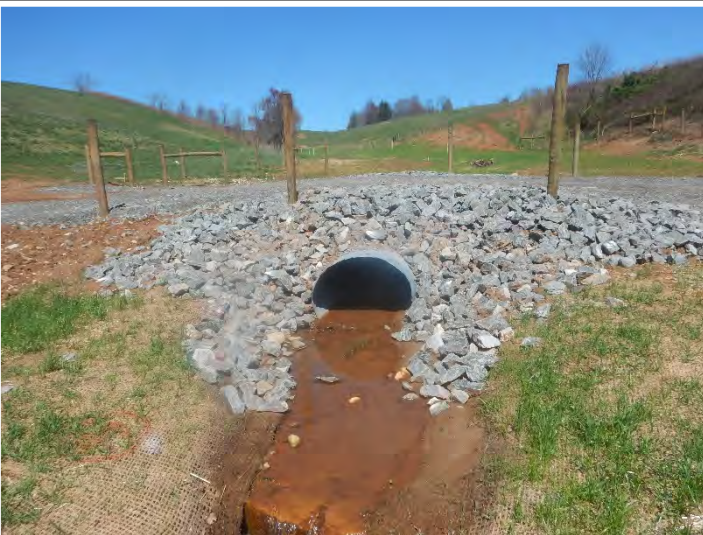
UT3 R3 - Looking Upstream (03/29/2021)
