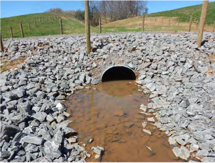
UT4 R3 - Looking Upstream (03/29/2021)
