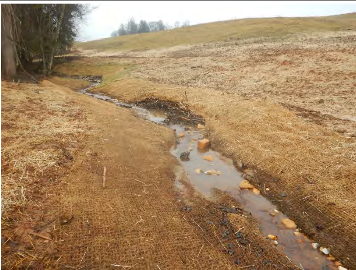
PHOTO POINT 21 UT3 R3 – upstream (01/25/2021)
