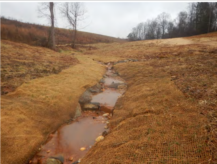
PHOTO POINT 18 UT3 R1 – upstream (01/25/2021)
