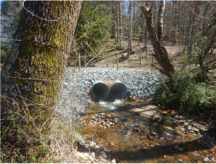
Hanks Branch R3 - Perched - Looking Upstream (03/29/2021)
