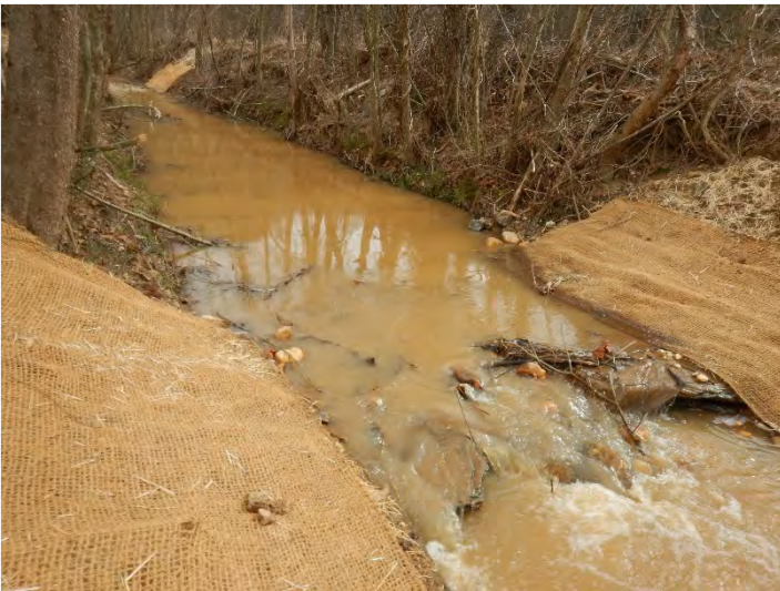
PHOTO POINT 11 Hank's Branch R3 – upstream (02/02/2021)
