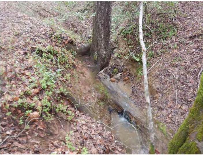
PHOTO POINT 31 UT5 R1 – upstream (3/24/2022)
