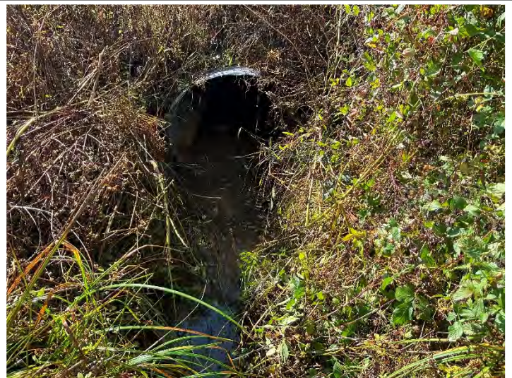
UT3 R3 - Looking Downstream (10/17/2022)
