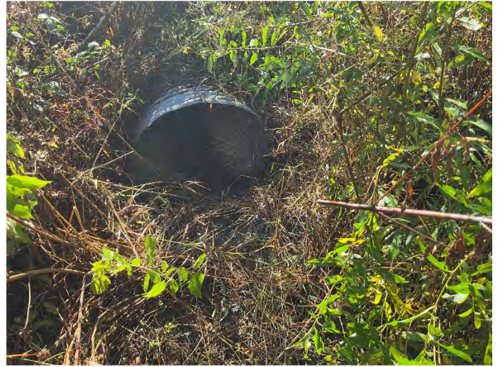
UT4 R3 - Looking Downstream (10/17/2022)
