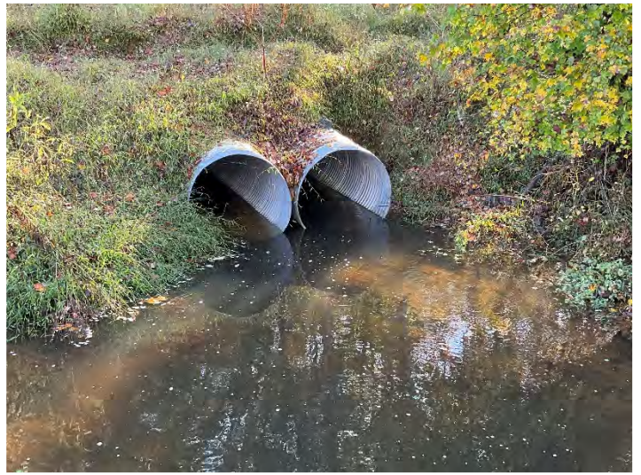
Hanks Branch R3 – Repaired Culvert Outlet (10/17/2022)
