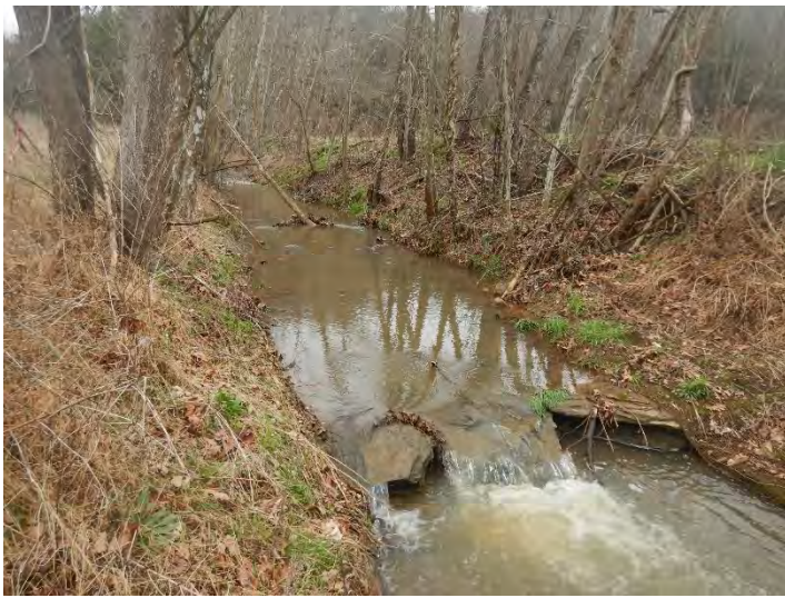
PHOTO POINT 11 Hank's Branch R3 – upstream (3/24/2022)
