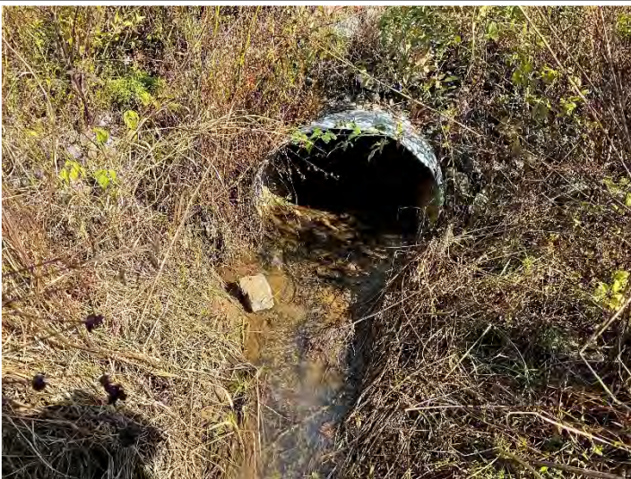
UT3 R3 - Looking Upstream (10/17/2022)
