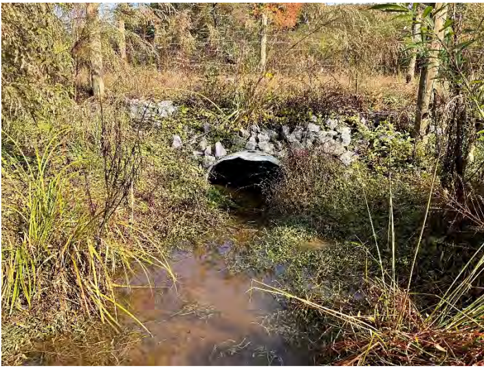
UT5 R2 - Looking Upstream (10/17/2022)
