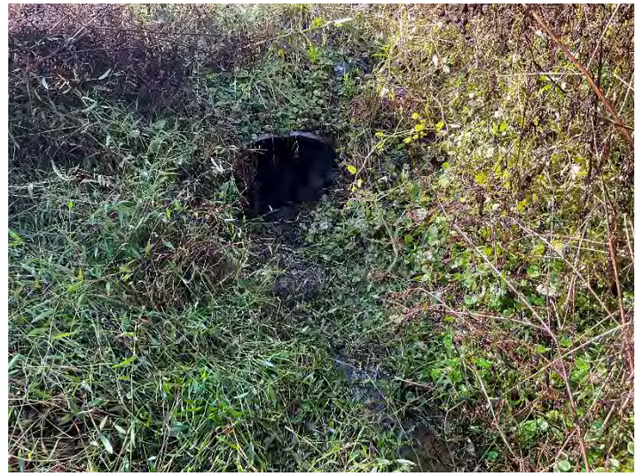
UT5 R2 - Looking Downstream (10/17/2022)
