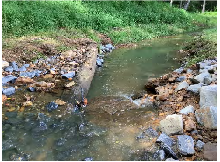
Hanks Branch R2 – Repaired J-Hook (8/17/2022)
