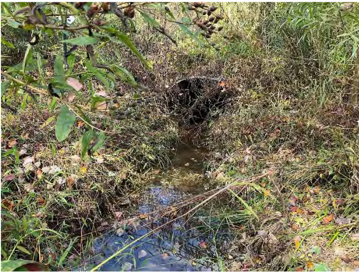
UT1 - Looking Upstream (10/17/2022)
