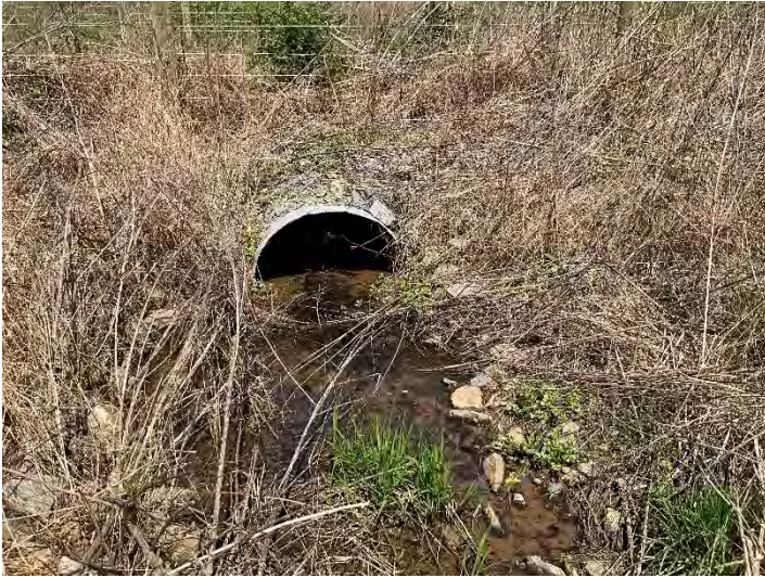
UT4 R3 - Looking Upstream (4/20/2023)
