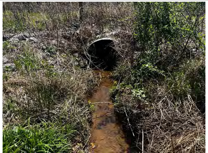
UT3 R3 - Looking Downstream (4/20/2023)
