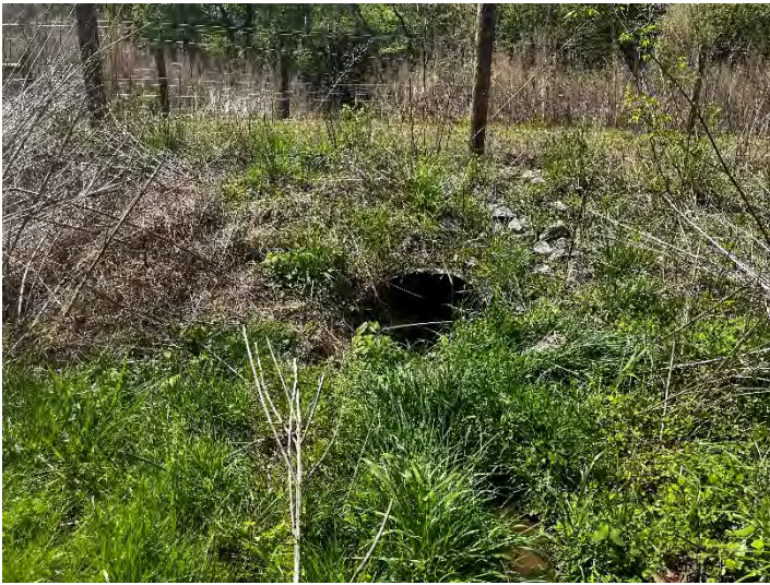
UT5 R2 - Looking Upstream (4/20/2023)
