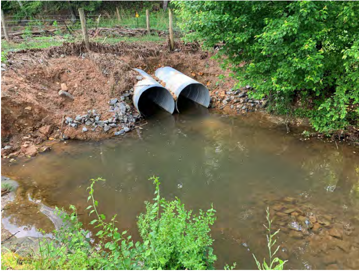
Hanks Branch R3 – Culvert Outlet (6/21/2023)
