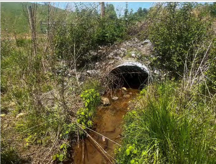
UT3 R3 - Looking Upstream (4/20/2023)
