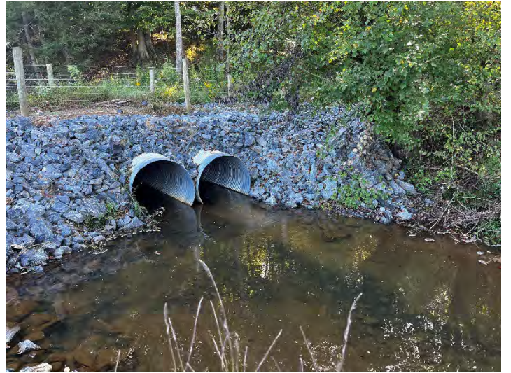
Hanks Branch R3 – Repaired Culvert Outlet (10/17/2023)
