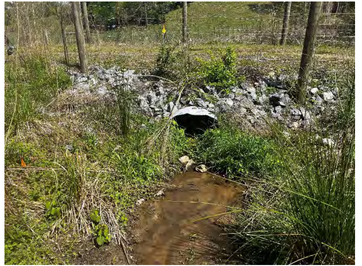
UT5 R2 - Looking Downstream (4/20/2023)
