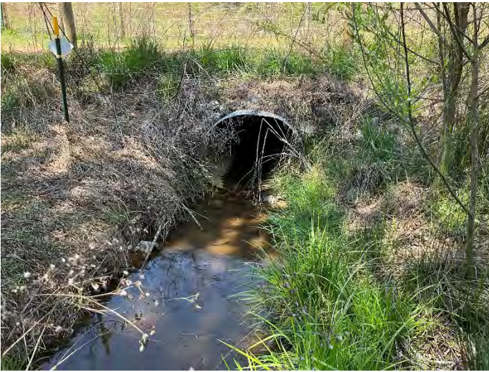
UT1 - Looking Upstream (4/20/2023)
