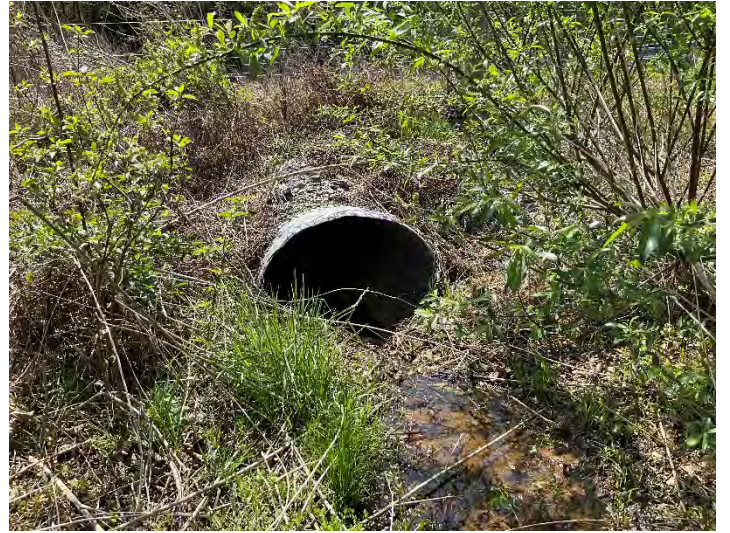
UT4 R3 - Looking Downstream (4/20/2023)
