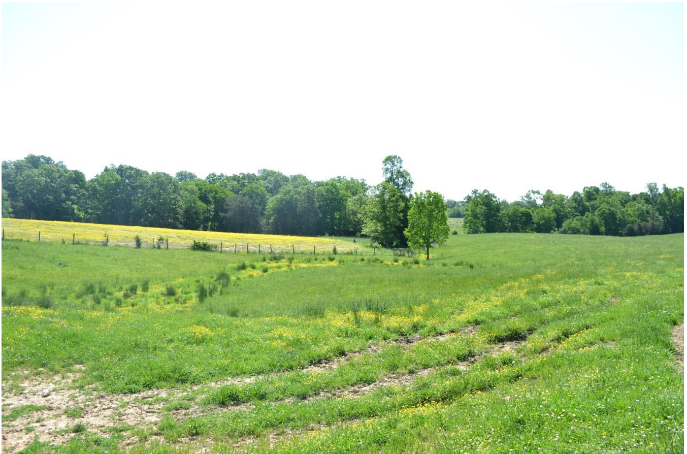
Adjacent to earthen dam along UT-1 looking downstream
