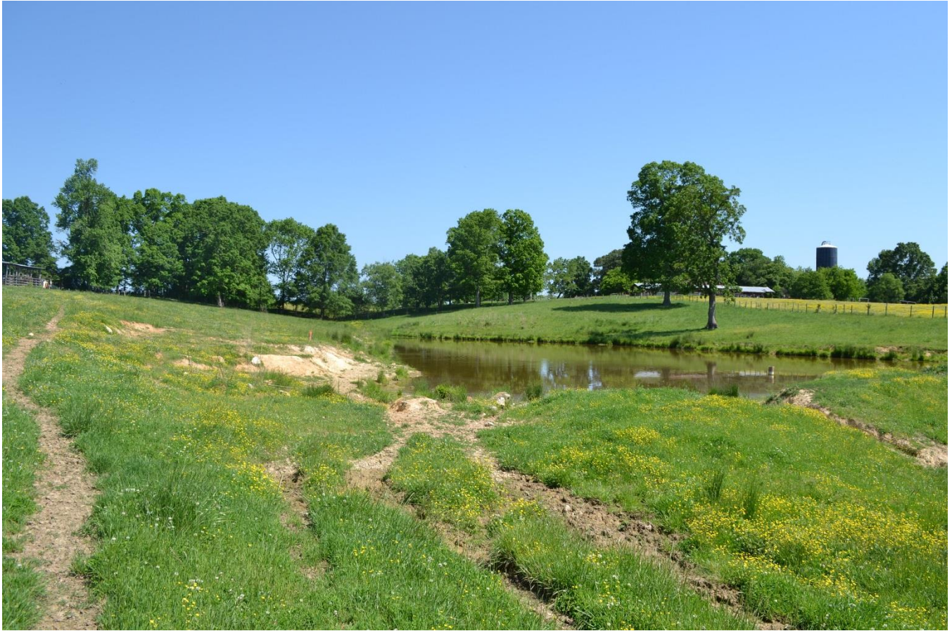
Earthen dam along UT-1 looking upstream
