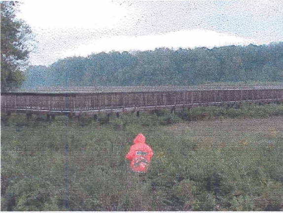
Photo 1: From SR 2833 looking Northeast
