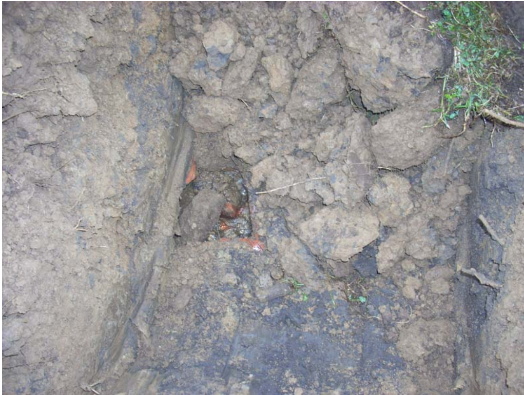
Photo 11: Test Pit TP-26
