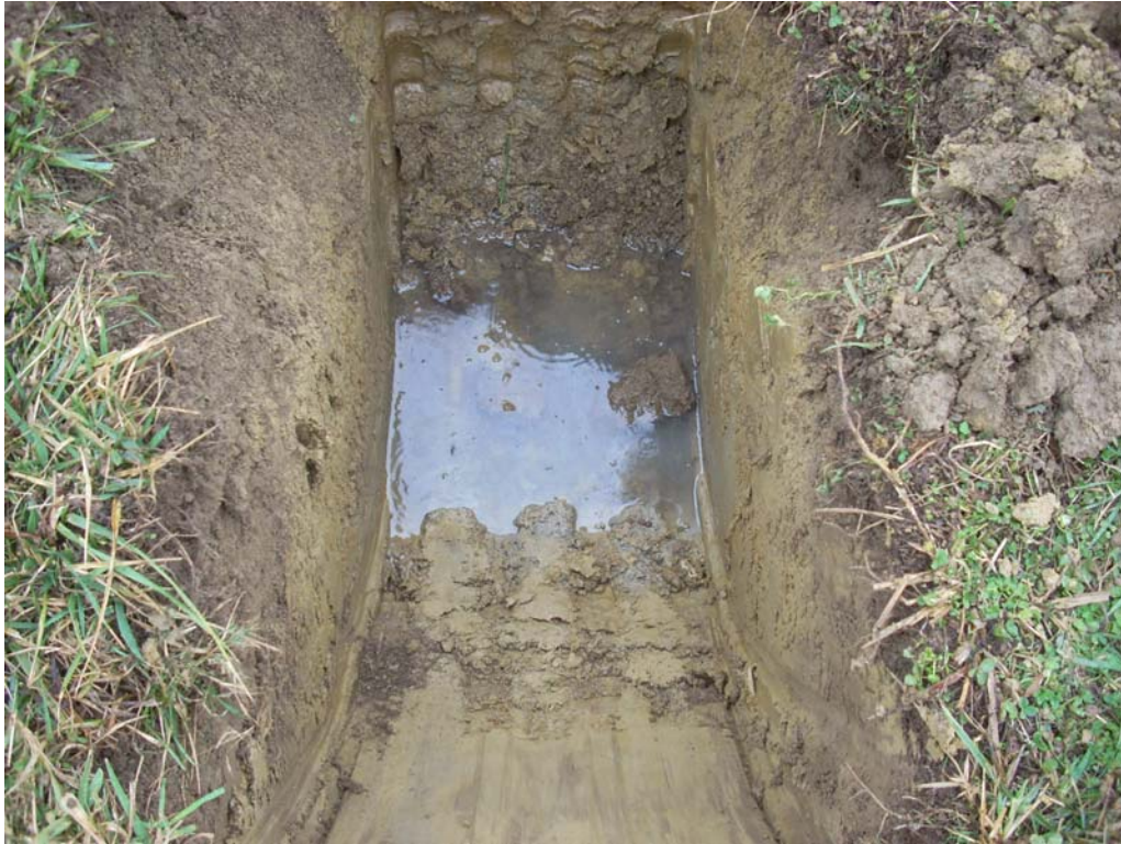
Photo 1: Test Pit TP-1
