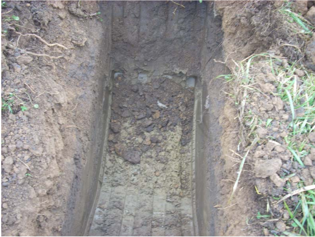
Photo 5: Test Pit TP-16
