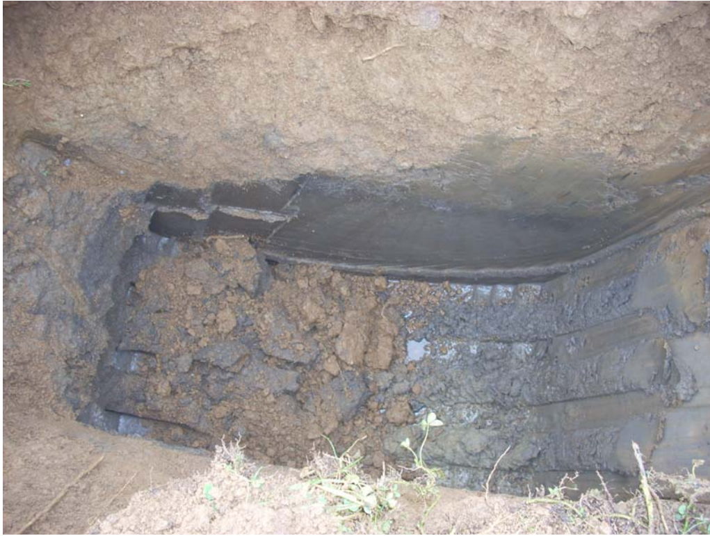
Photo 7: Test Pit TP-17
