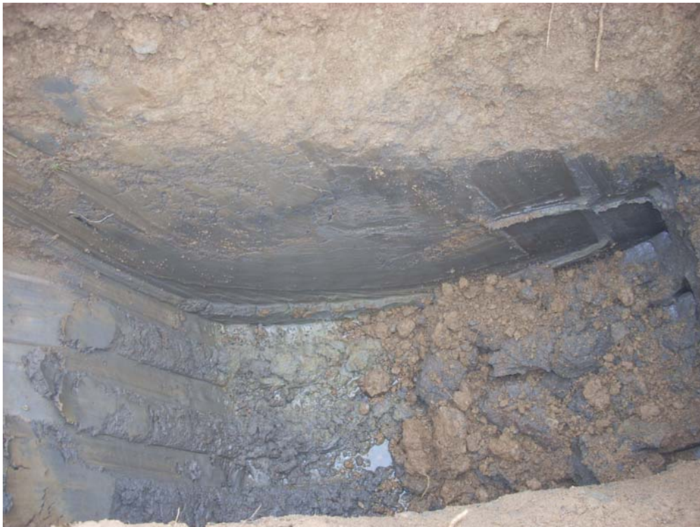
Photo 8: Test Pit TP-17
