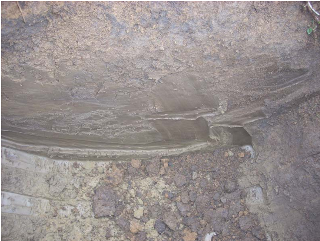
Photo 6: Test Pit TP-16
