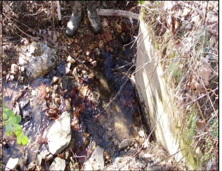
MC-UT1 makes a 90° turn into this box culvert near the barn.
