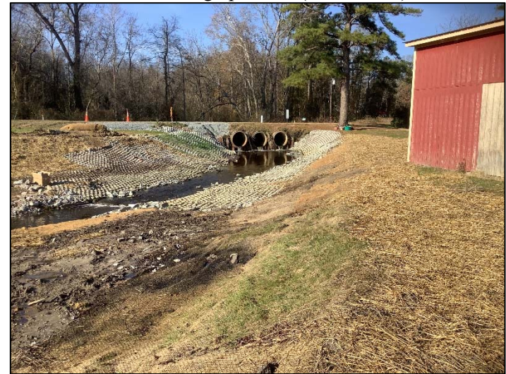
Plunge pool and boulder toe protection below NC-96 culvert on RL1-A (12/15/2020)
