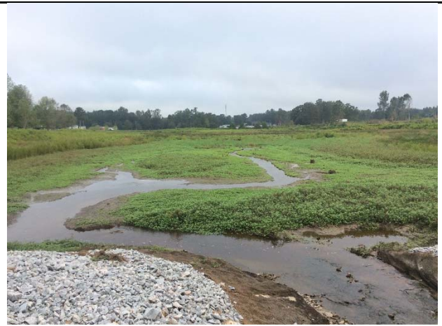
Pond Footprint – Looking Upstream (9/25/2018)
