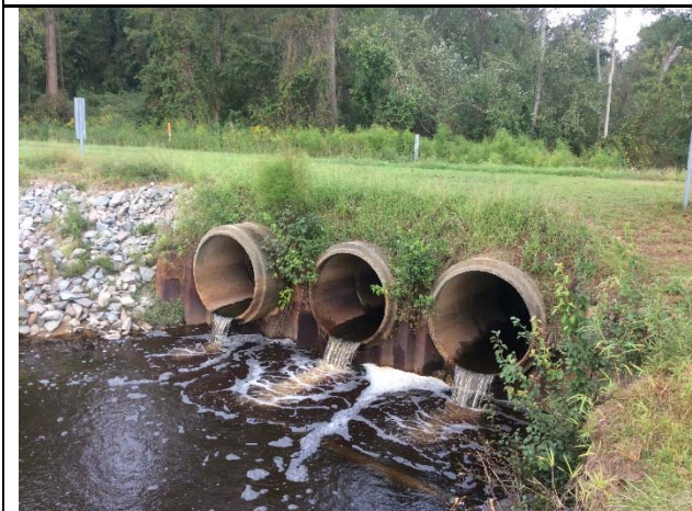
Culverts – Top of Project at NC-96 (9/25/2018)
