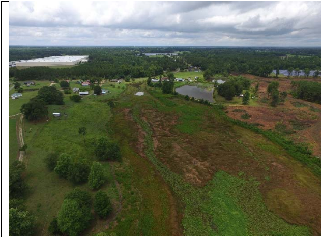
Pond Footprint – Looking Upstream (7/30/2018)
