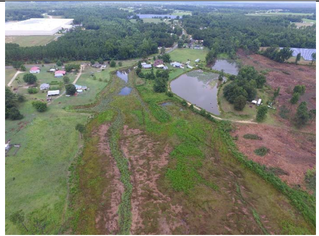
Pond Footprint – Looking Upstream (7/30/2018)
