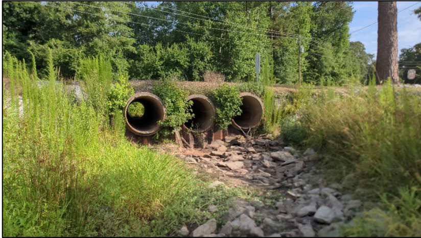
Plunge pool and boulder toe protection below NC-96 culvert on RL1-A (06/28/2022)
