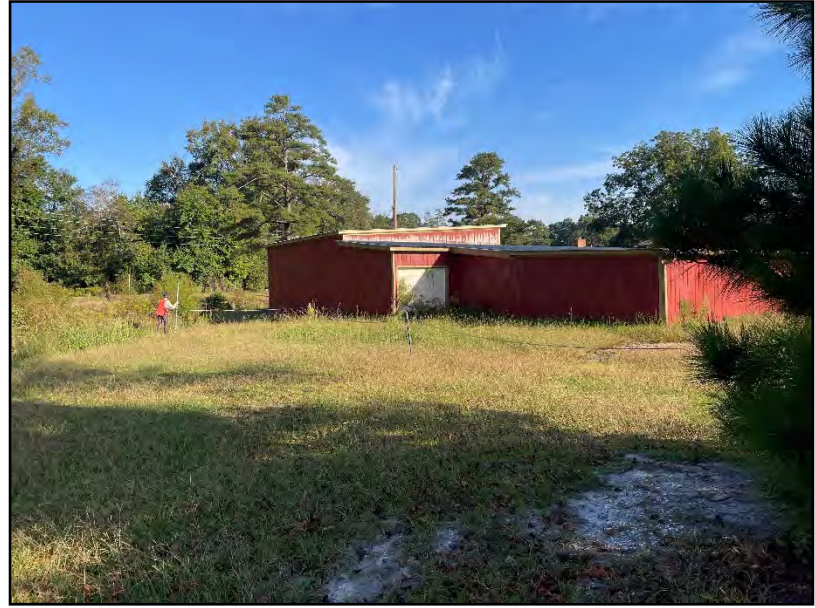
Markers added to Northern Encroachment (7/27/2023)
