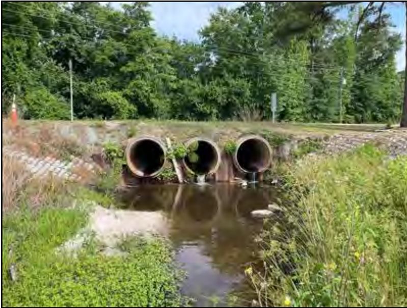
Plunge pool and boulder toe protection below NC-96 culvert on RL1-A (05/18/2023)
