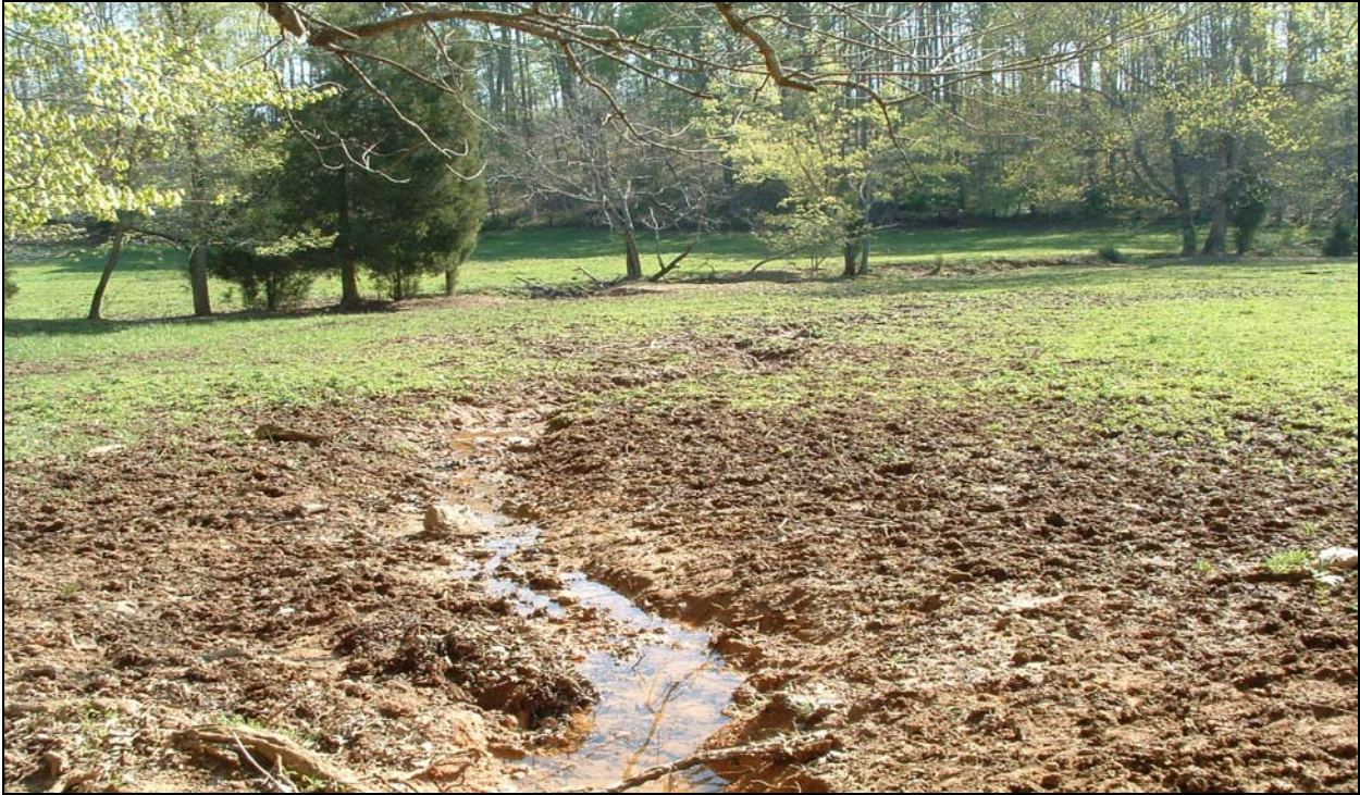
Photograph 27 – A portion of the flow in UT3 crosses a field towards the right bank of UTBC. The channel appears to be newly formed, either due to overbank flow or was excavated to redirect flow.
