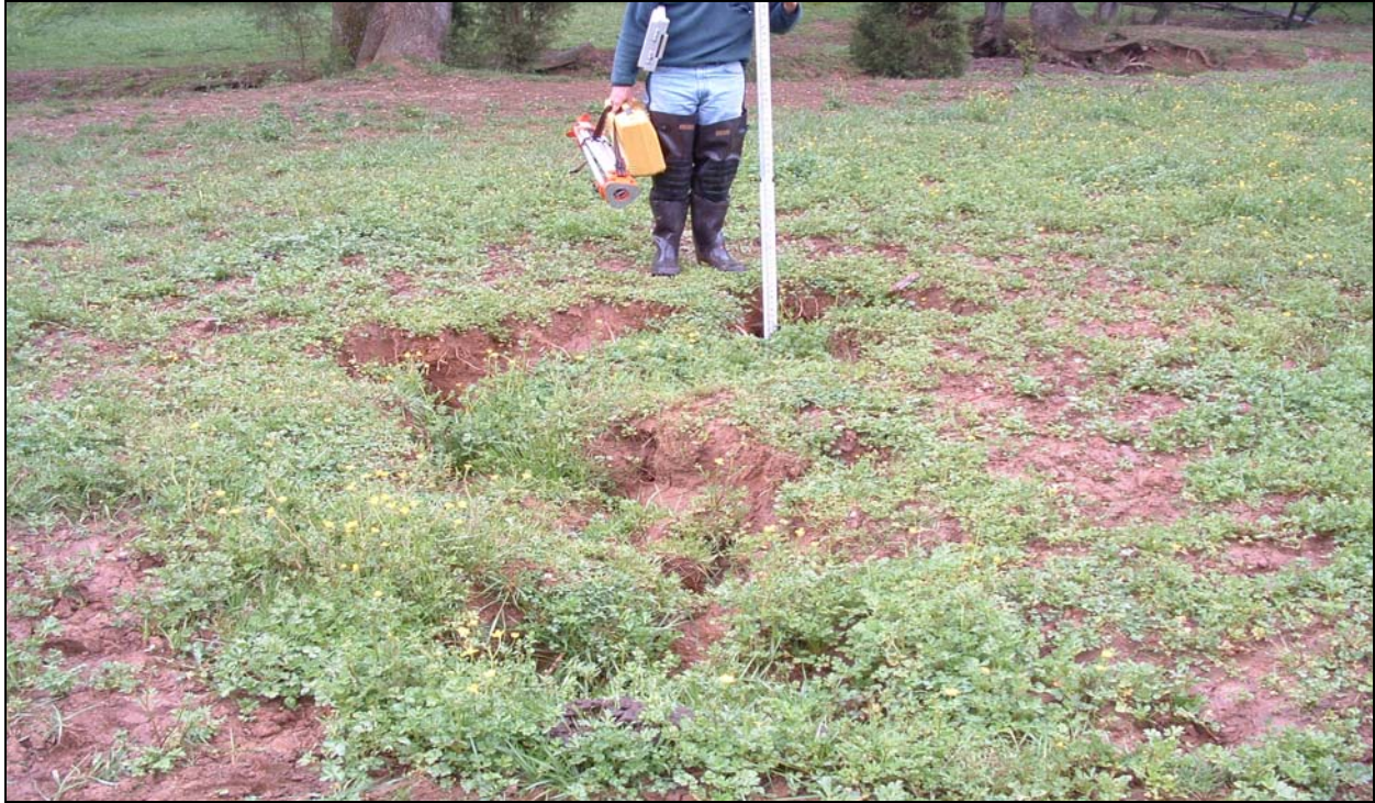
Photograph 33 – Sinkholes in riparian area approximately 30 feet from right bank of UTBC. Maximum depth is approximately two feet.
