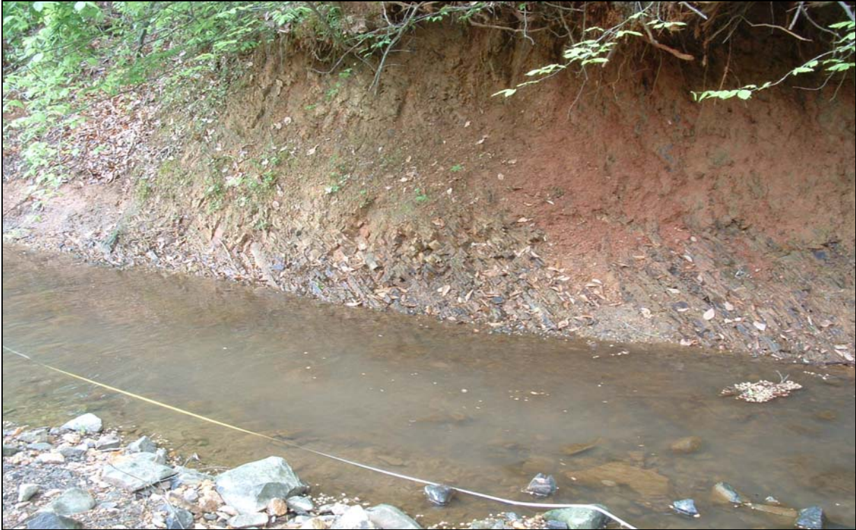
Photograph 3 – Weathered bedrock along right bank and in UTBC streambed (Station 10+20 to 10+35).
