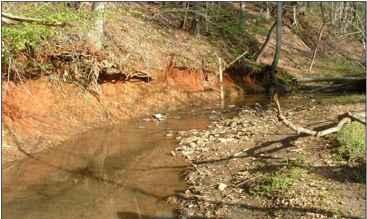
Photograph 2 – View looking upstream at top of project site. Logs in stream in upper right of photo mark station 10+00. Scour along the right bank is predominantly into weathered bedrock.
