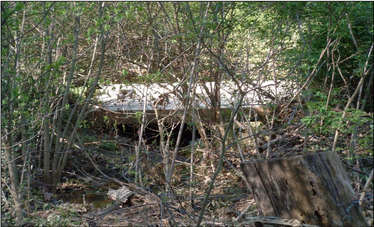
Photograph 40 – Concrete slab crossing stream channel approximately 20 feet downstream of project boundary.
