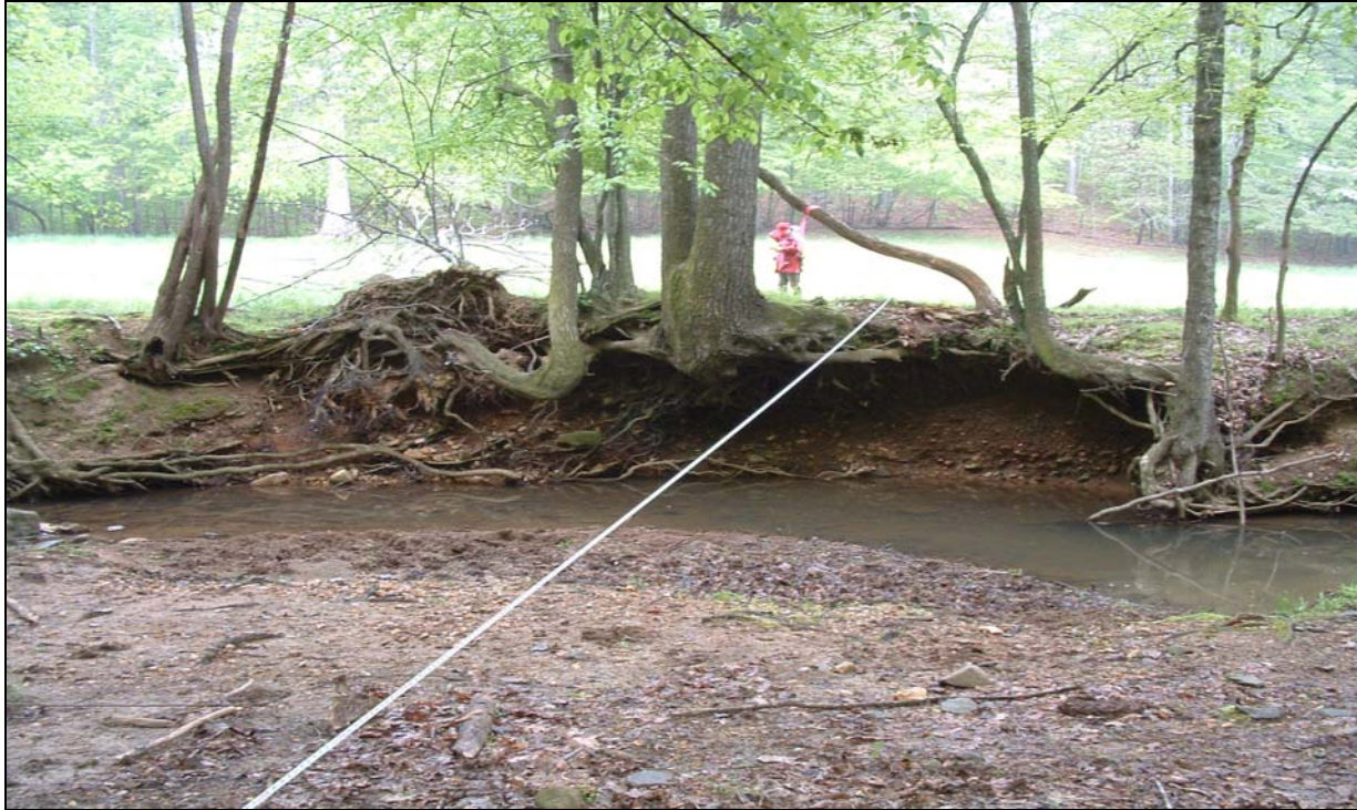
Photograph 7 – Undercut left bank at Cross-section 2, top of bank overhangs ~2.3 feet.
