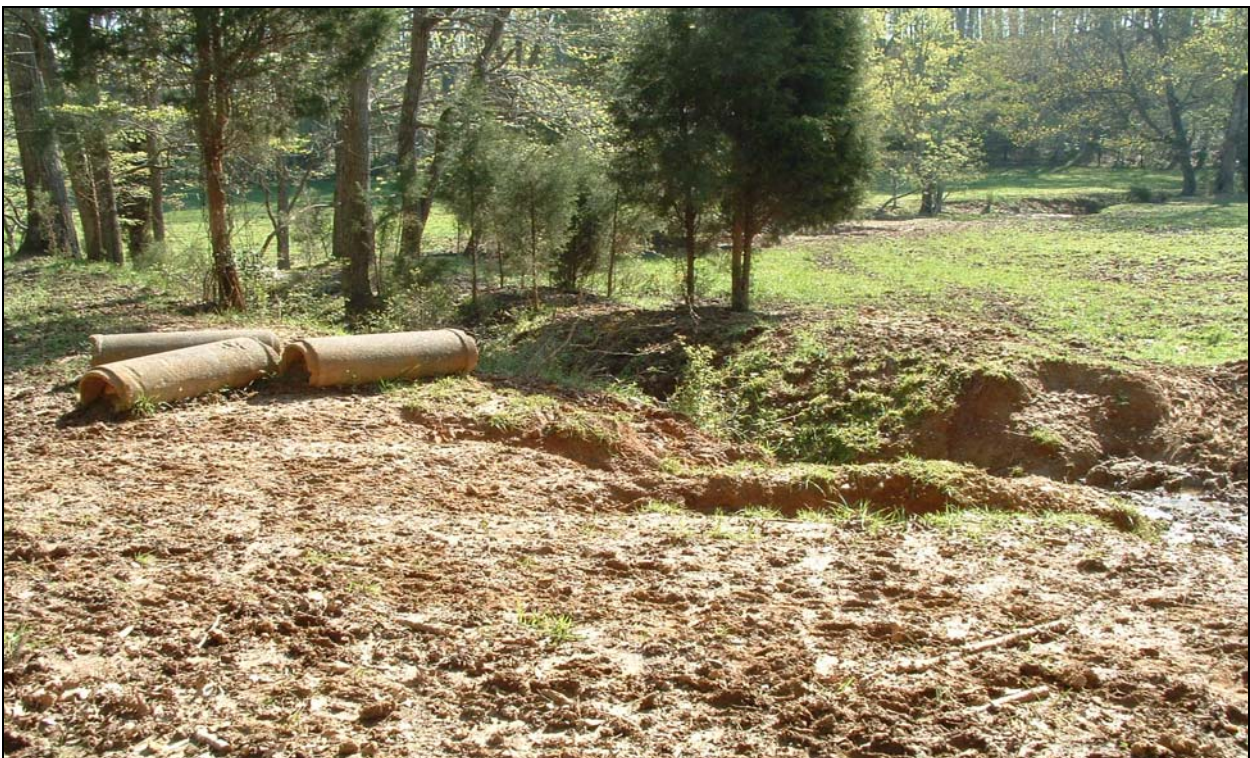
Photograph 26 – Concrete pipe along UT3, above headcut.
