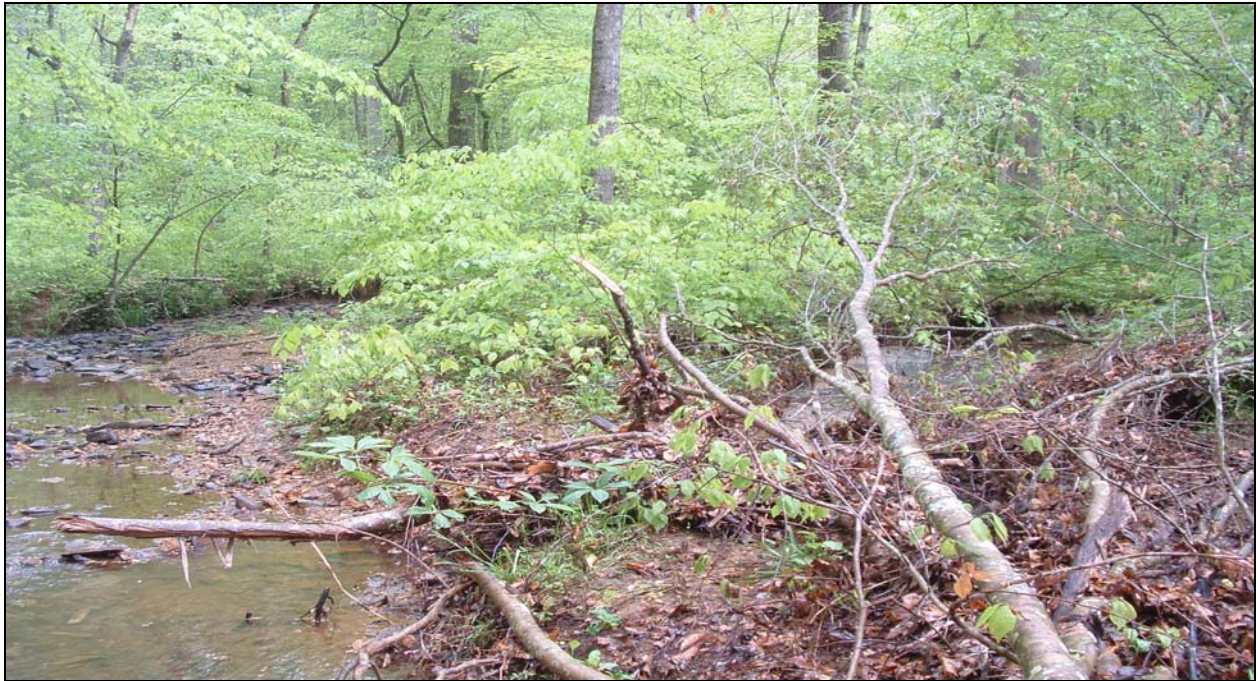
Photograph 1 – View of UTBC prior to entering project site, looking upstream from Station 10+00 across the McCain property boundary.
