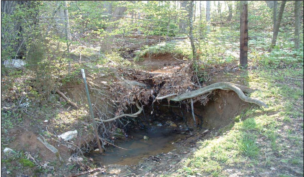
Photograph 16 – Headcut along Trib 2 at property boundary, approximately 50 feet upstream from confluence with UTBC.
