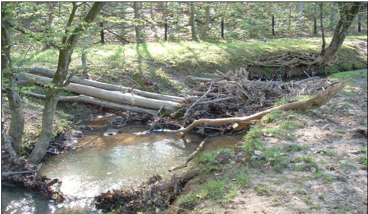
Photograph 34 – View downstream of series of debris jams. The disruption of flow has caused localized bank erosion and the formation of plunge pools. Fence line approximately 20 feet from left top of bank marks property boundary.
