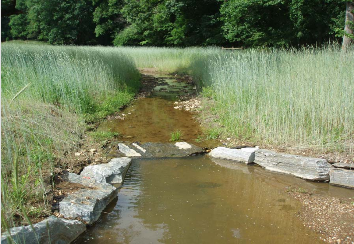
Photo Point 9u: View looking upstream near Station 30+30. 5/29/09 – As-Built
