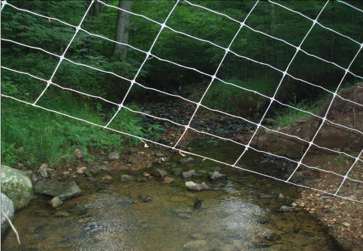
Photo Point 1u: View looking immediately upstream of the project. 5/29/08 – As-Built
