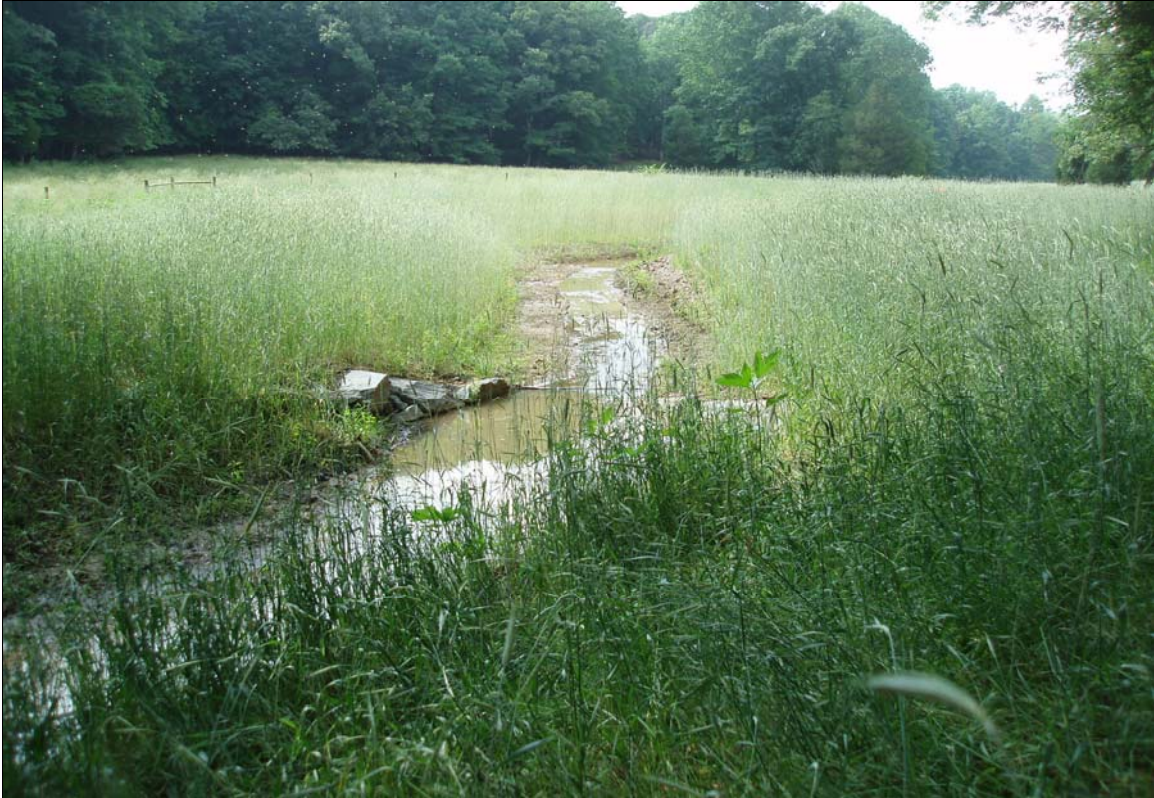
Photo Point 10u: View looking upstream near Station 34+25. 5/29/09 – As-Built
