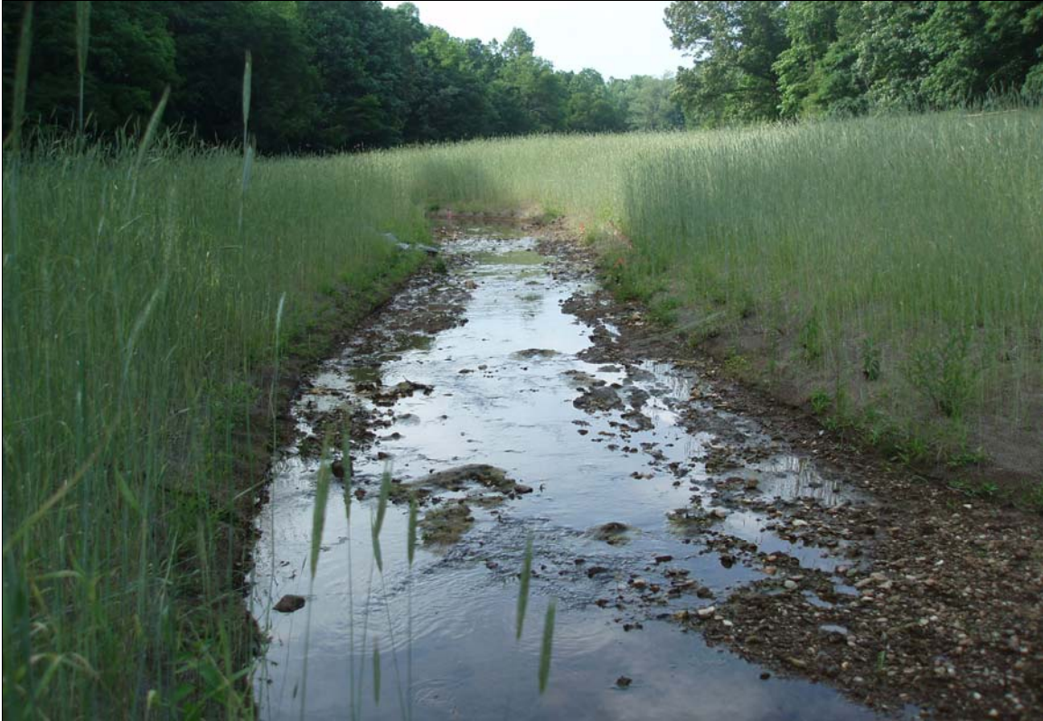
Photo Point 8u: View looking upstream near Station 27+75. 5/29/09 – As-Built
