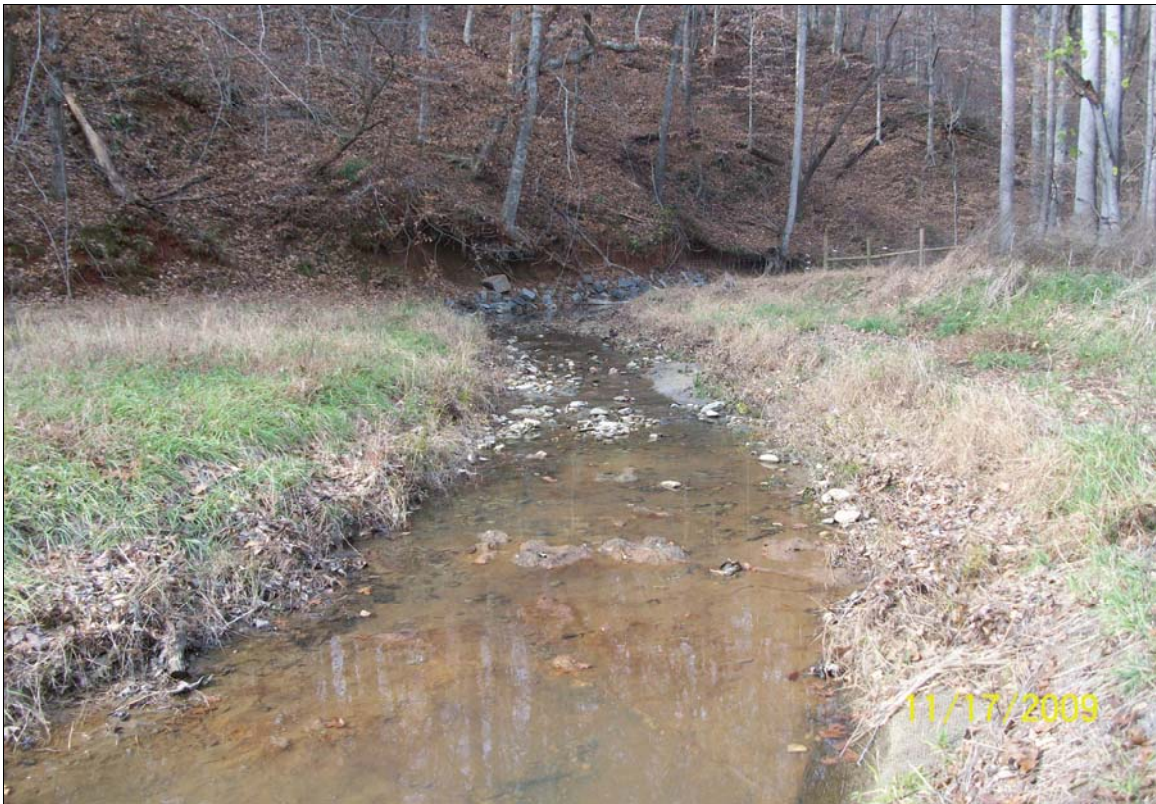
Photo Point 2u: View looking upstream taken near Station 11+50. 11/17/09 – MY-01
