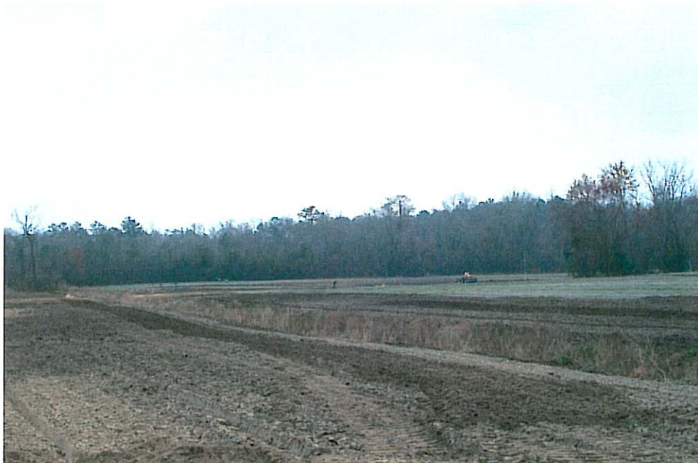
↓ View of site preparation prior to planting
