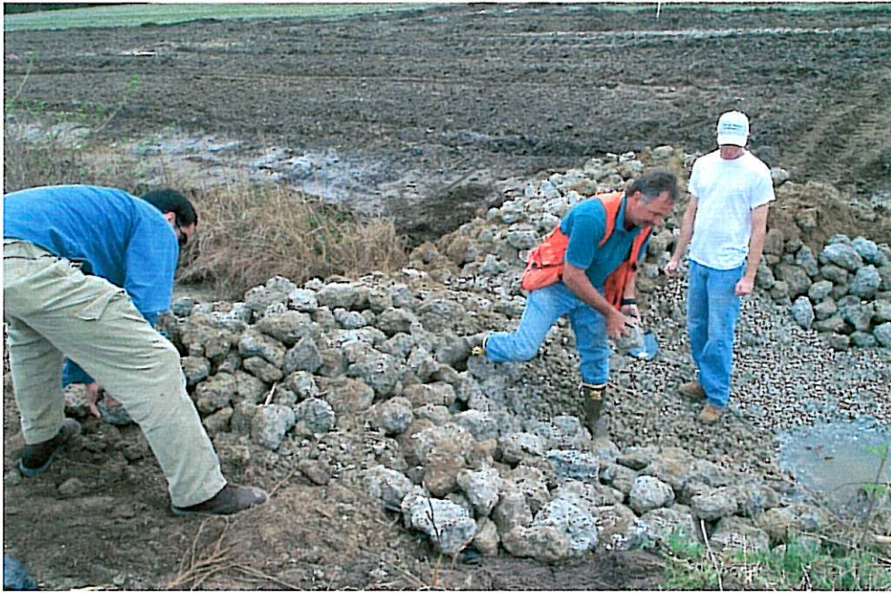
↓ Installation of check dam during project construction (February 2003)
