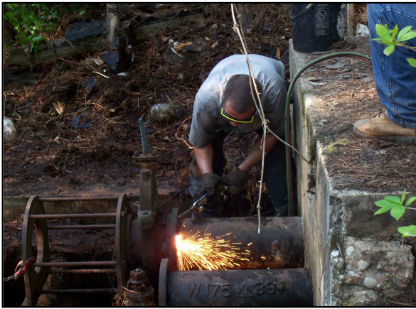
Photo 7: Removal of two gate valves using an acetylene torch.
