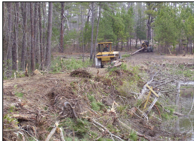
Photo 9: Grapple skidder (background) and bull dozer (foreground) working in tandem to remove trees from the former dam.
