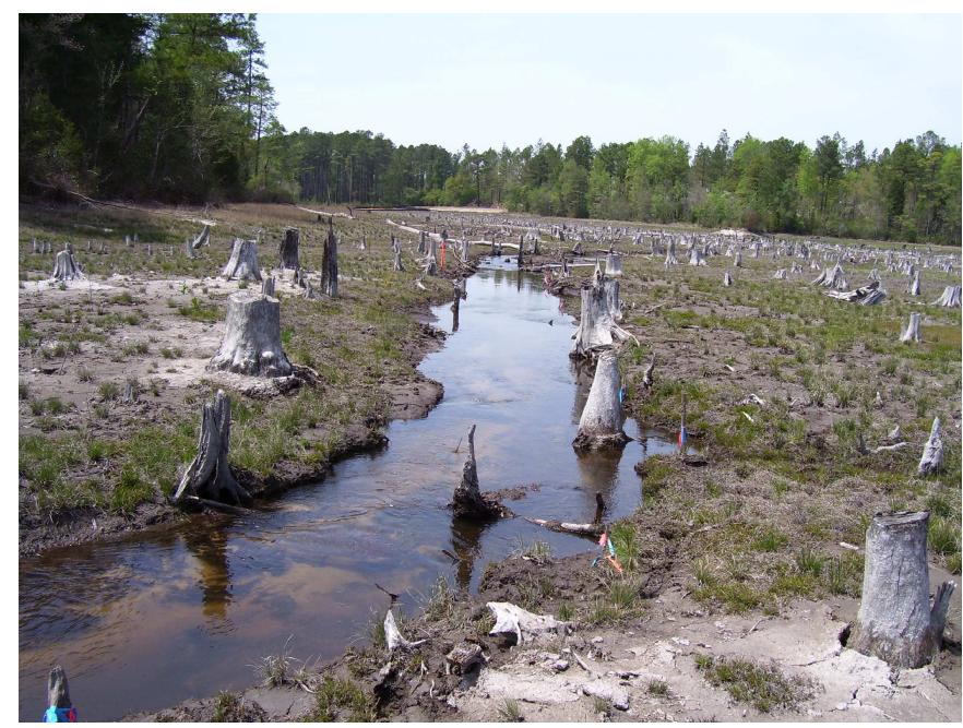
Reach 3 Cross-Section upstream looking downstream
