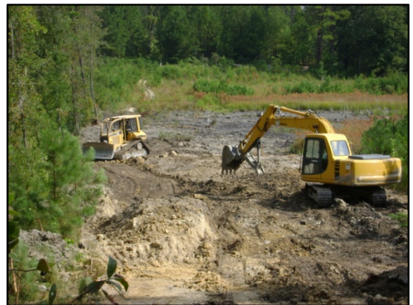
Grading the former dam surface
