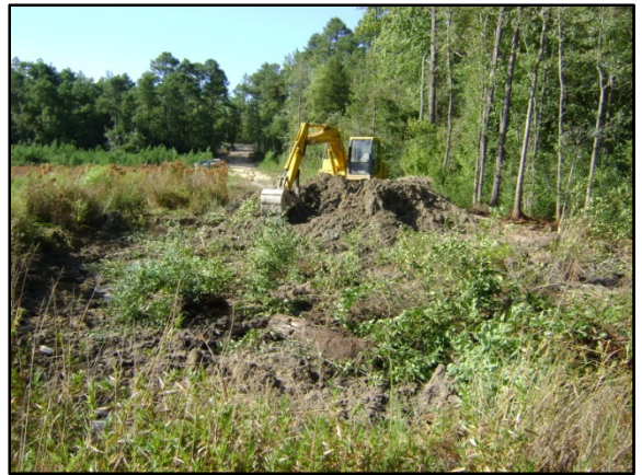
Removing beaver dam and beginning grading activities
