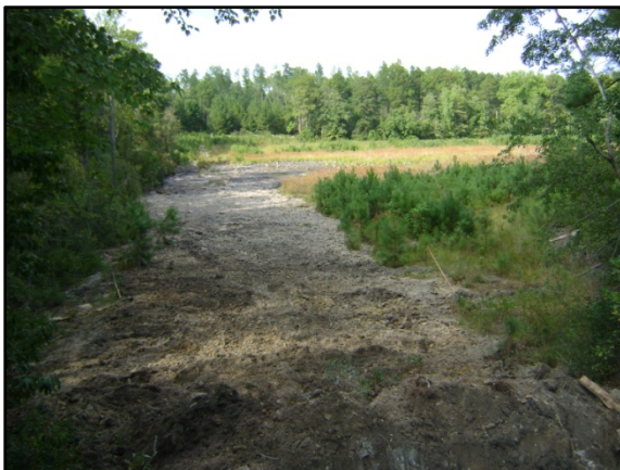
Finished grade of former dam from southern Site boundary
