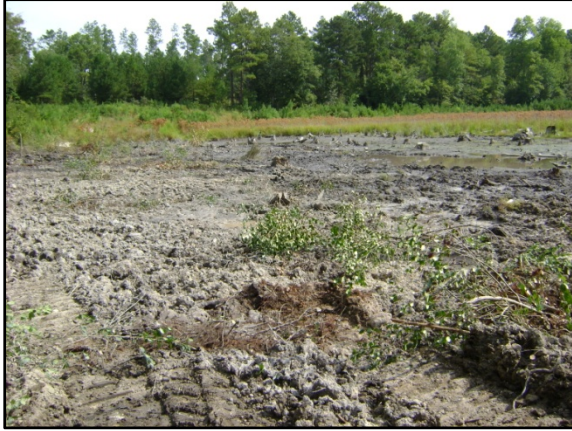
Following grading, the former dam elevation now matches the surrounding floodplain
