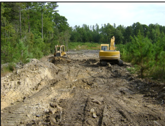
Grading the former dam surface
