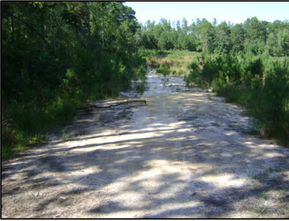
Dam surface prior to grading activities
