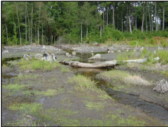
Confluence of existing channel with newly reshaped channel
