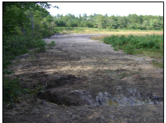
Trench and soil pile at southern Site boundary
