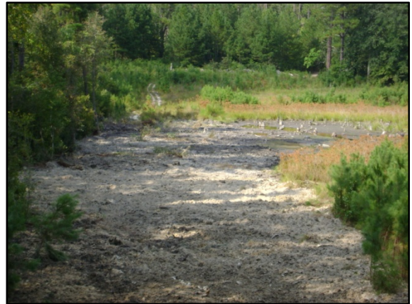
Finished grade near wetland boundary
