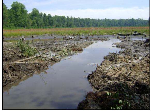
Stream channel flowing through newly graded area
