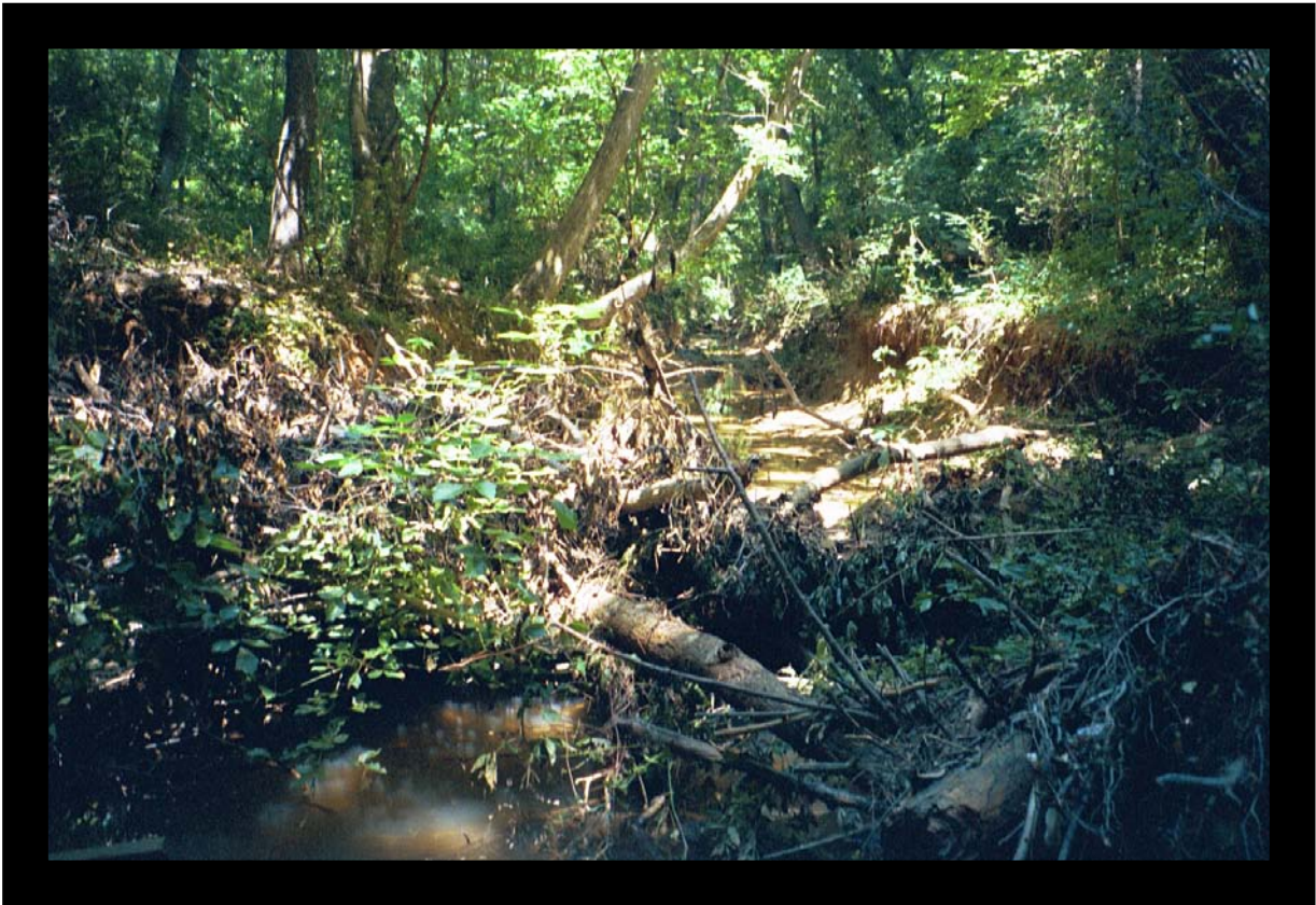
Photo 3: View of debris jam, near Station 14+75. Numerous debris jams exist throughout the project reach, as a result of fallen trees caused by bank erosion.
