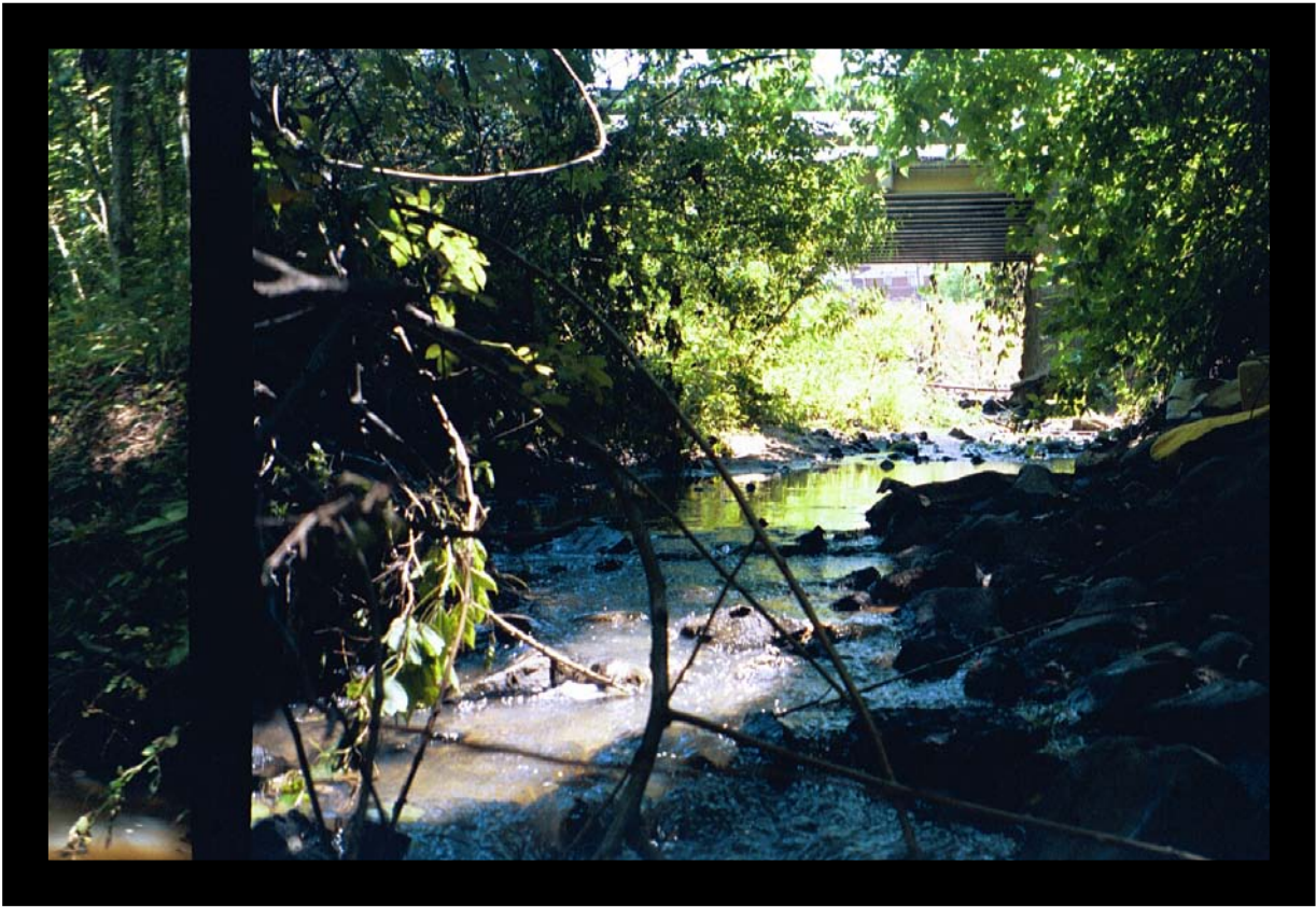
Photo 1: View of McIntyre Creek looking upstream at the Beatties Ford Bridge.
