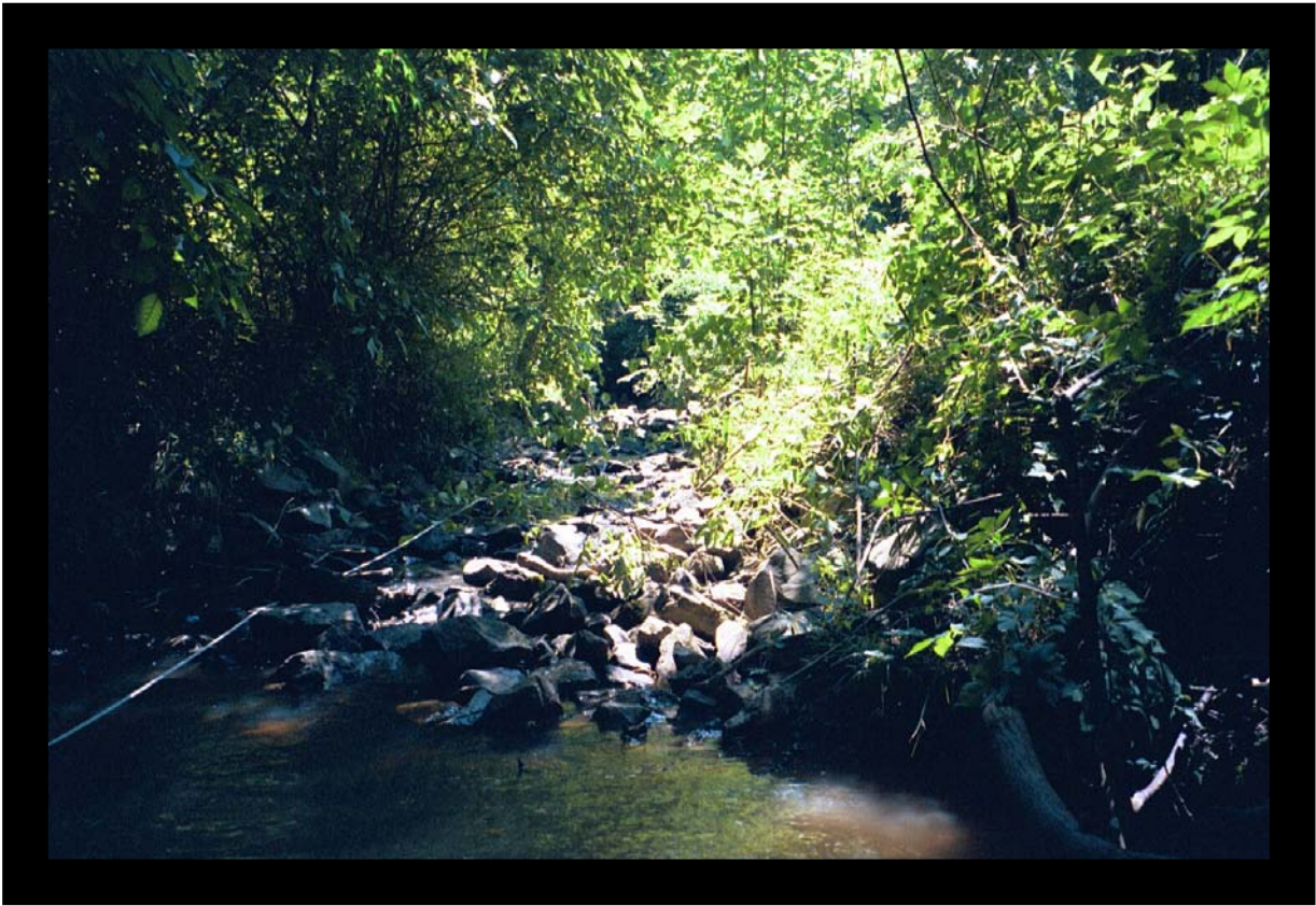
Photo 9: Rip rap channel extending downstream from gas pipeline crossing. This point divides the project reach into upper/lower portions.
