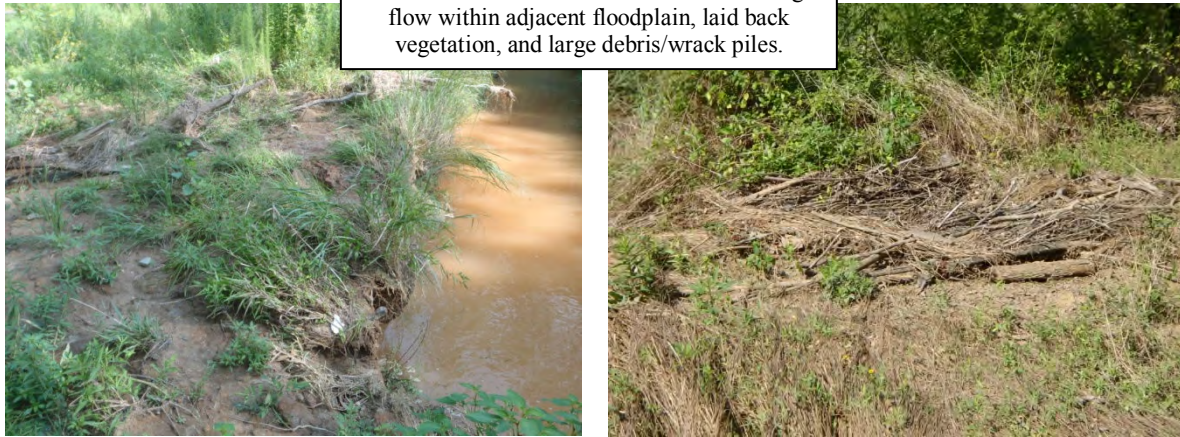
Photo 3: Evidence of overbank including laid back vegetation and recent standing water within the floodplain.
