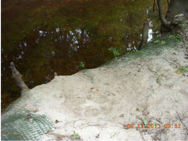
Photo 13. Sediment at berm cut
