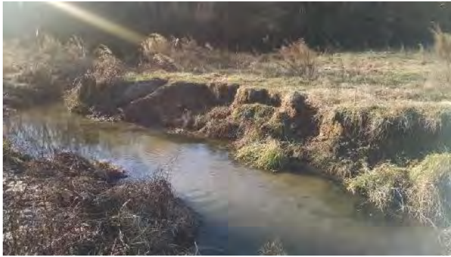
Vertical bank on the downstream portion of R3. Channel incision and mass wasting are visible.
