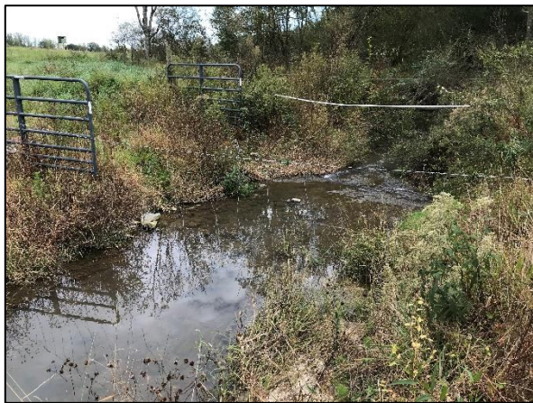
Stream crossing fence repairs near Sta. 38+00 facing downstream (3/11/2021)
