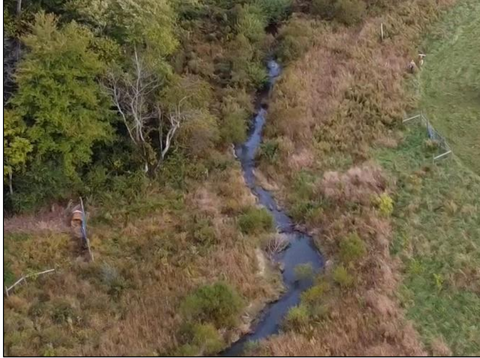
Stream crossing on Meadow Brook Reach 2, near Sta. 33+00 facing downstream (10/21/2021)
