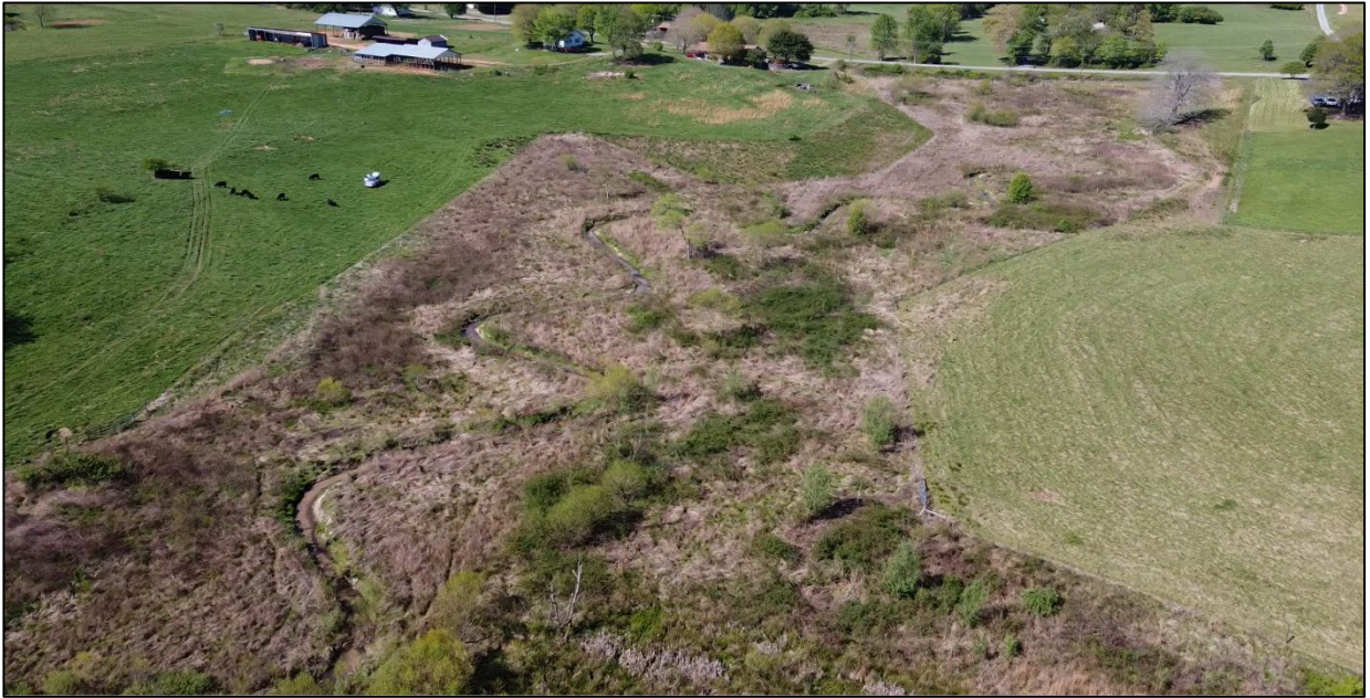
Site Overview Facing East (4/14/2023)
