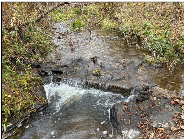
Representative Photo, Reach 1 Offset rock vane, facing Upstream (10/31/2023)
