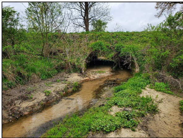
Photo Point 17 – Reach 1, Sta. 10+50 Facing Upstream (04/05/2023)
