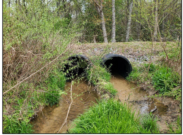
Photo Point 20 – UT, Sta 10+20 Facing Upstream (04/05/2023)
