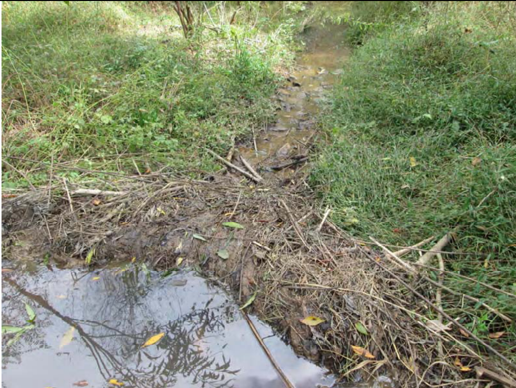
SP5: Beaver dam on lower M1 (STA 31+965) Taken: 10-18-2012
