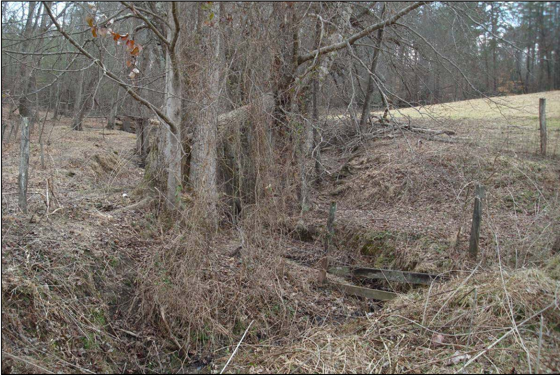
Sprouse Branch transition from woods to ag ditch @ Sta 201+00 facing upstream 2/18/11
