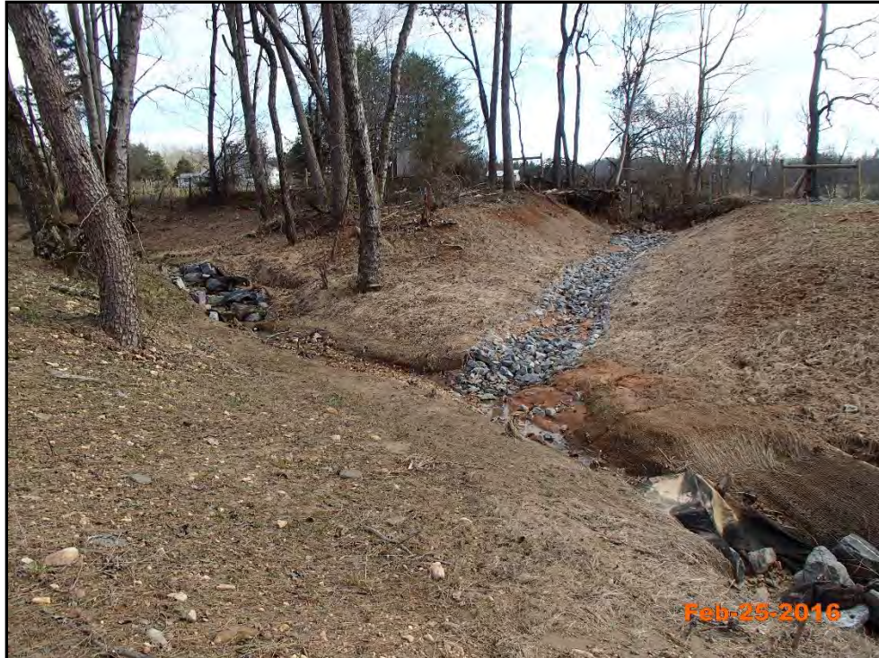
Upper Iva Branch – Permanent Photo Station 19 Station 303+75 - Looking Upstream
