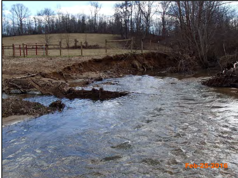
South Muddy Creek – Permanent Photo Station 8 Station 101+50 - Looking Upstream
