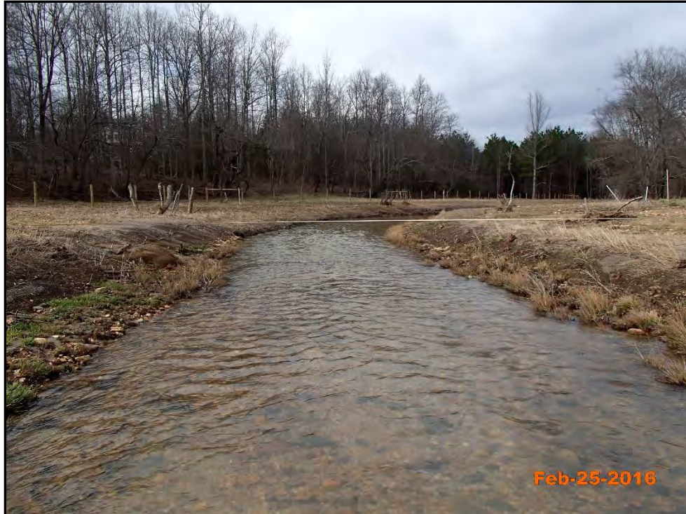
South Muddy Creek – Permanent Photo Station 11 Station 107+45 - Looking Downstream at Cross-Section 5
