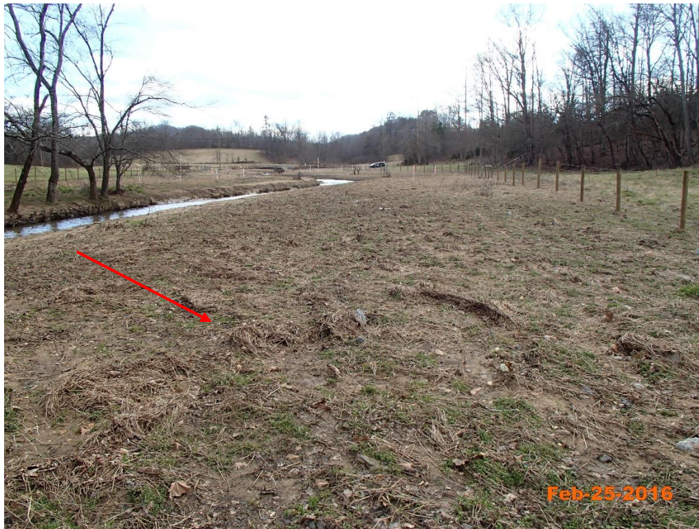
Photo #1 - South Muddy Creek Wrack Lines
