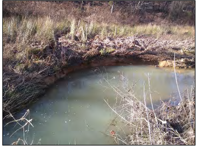
Outer bend erosion, Sta 46+25, 12/18/20
