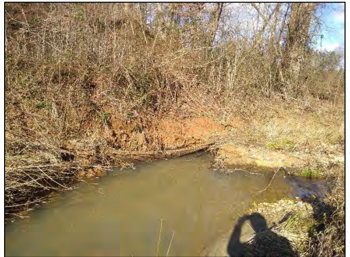
Outer bend erosion, Sta 54+25, 12/18/20
