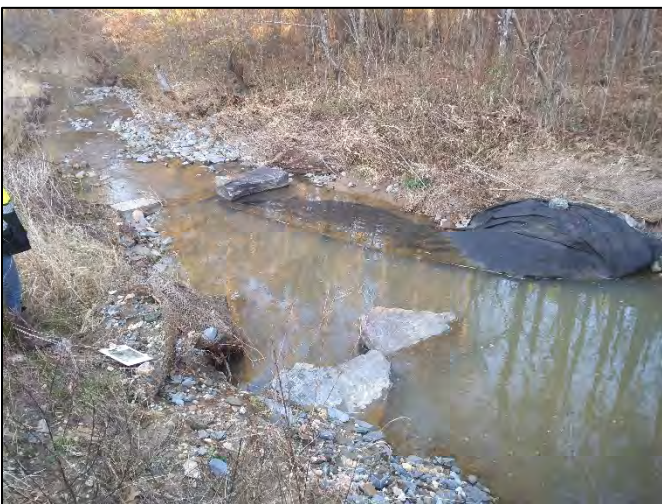
Damaged boulder sill, Sta 55+60, 12/18/20
