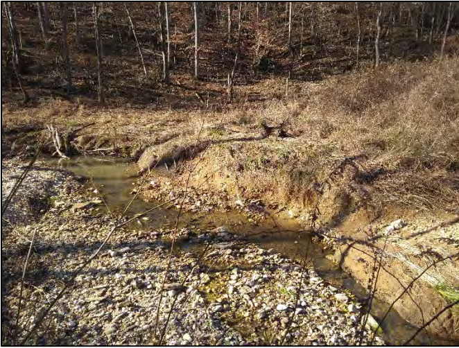
Outer bend erosion, Sta 39+50, 12/18/20
