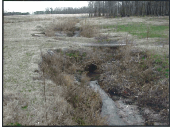
Looking downstream on Upper Reach of Main UT.
