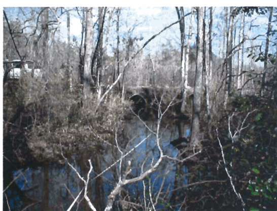
Looking upstream at culvert.
