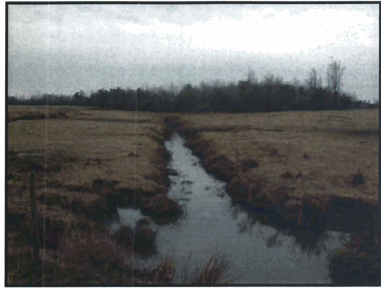
Looking upstream from access road on Main
