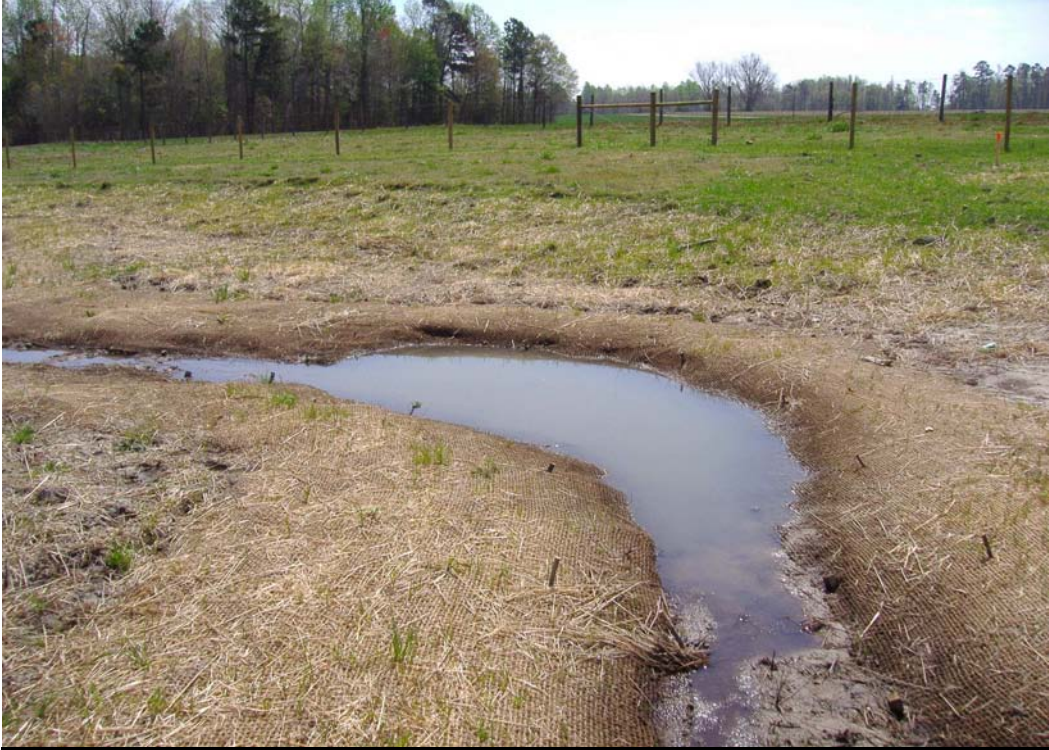
Photo of Cross-Section 2 - Looking Downstream @ STA 2+50
