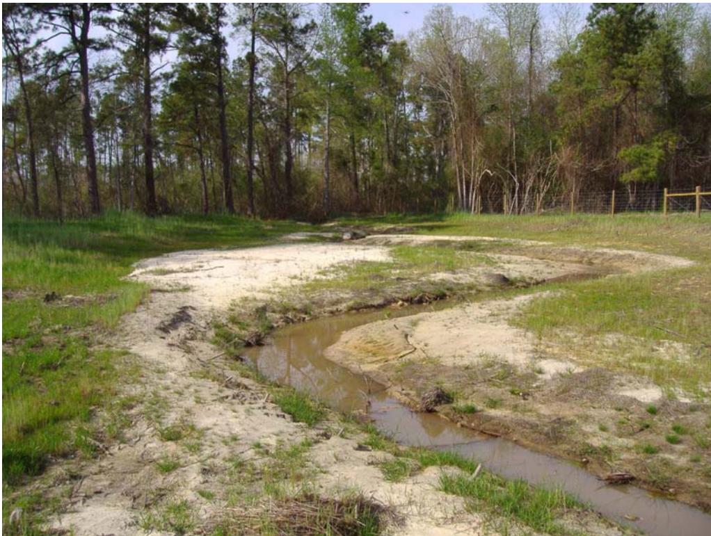
Photo Station 32. Pool Cross-section 8 – Downstream – Lower Reach
