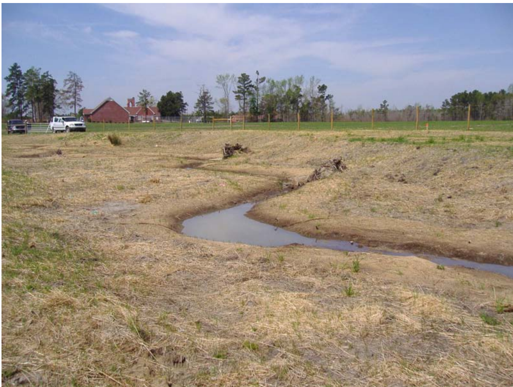
Photo Station 6. Pool Cross-section 2 – Upstream – Western Reach
