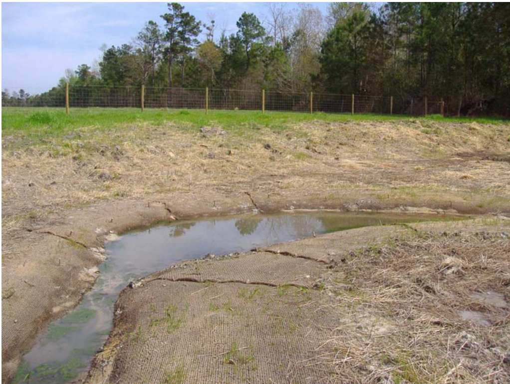
Photo Station 12. Pool Cross-section 3 – Upstream – Upper Reach
