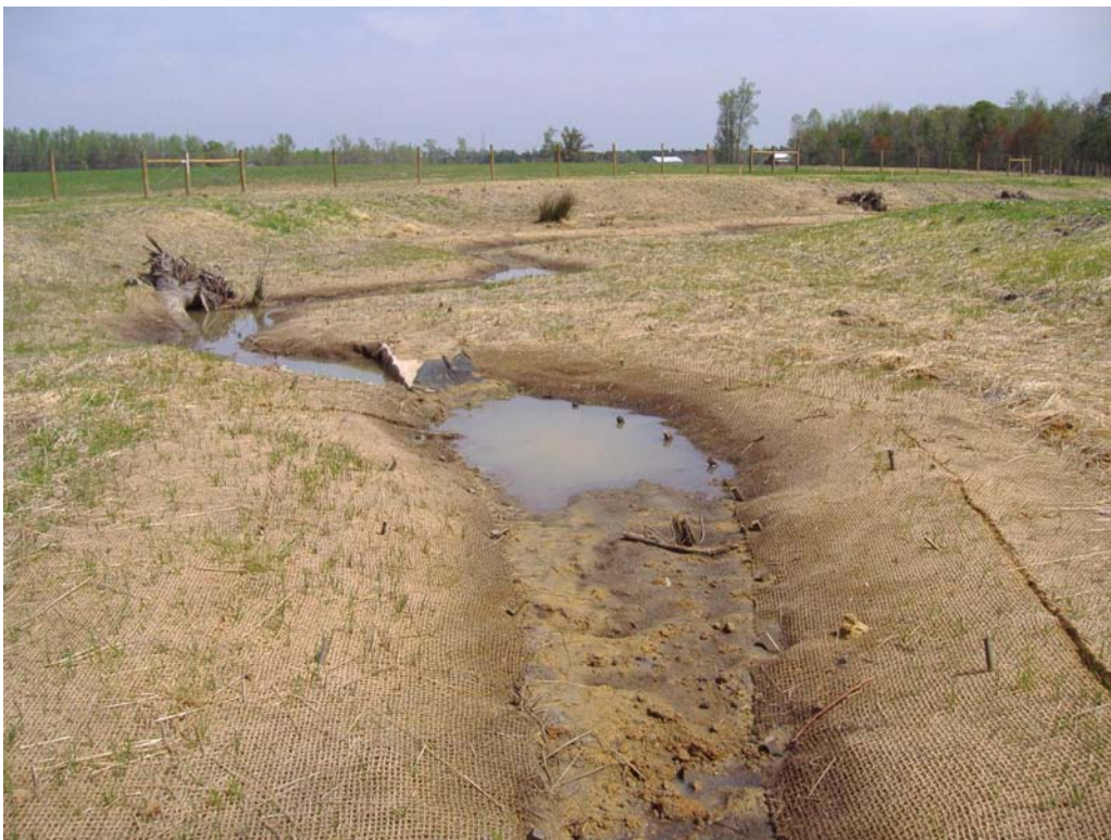
Photo Station 2. Beginning of Western Reach – Downstream
