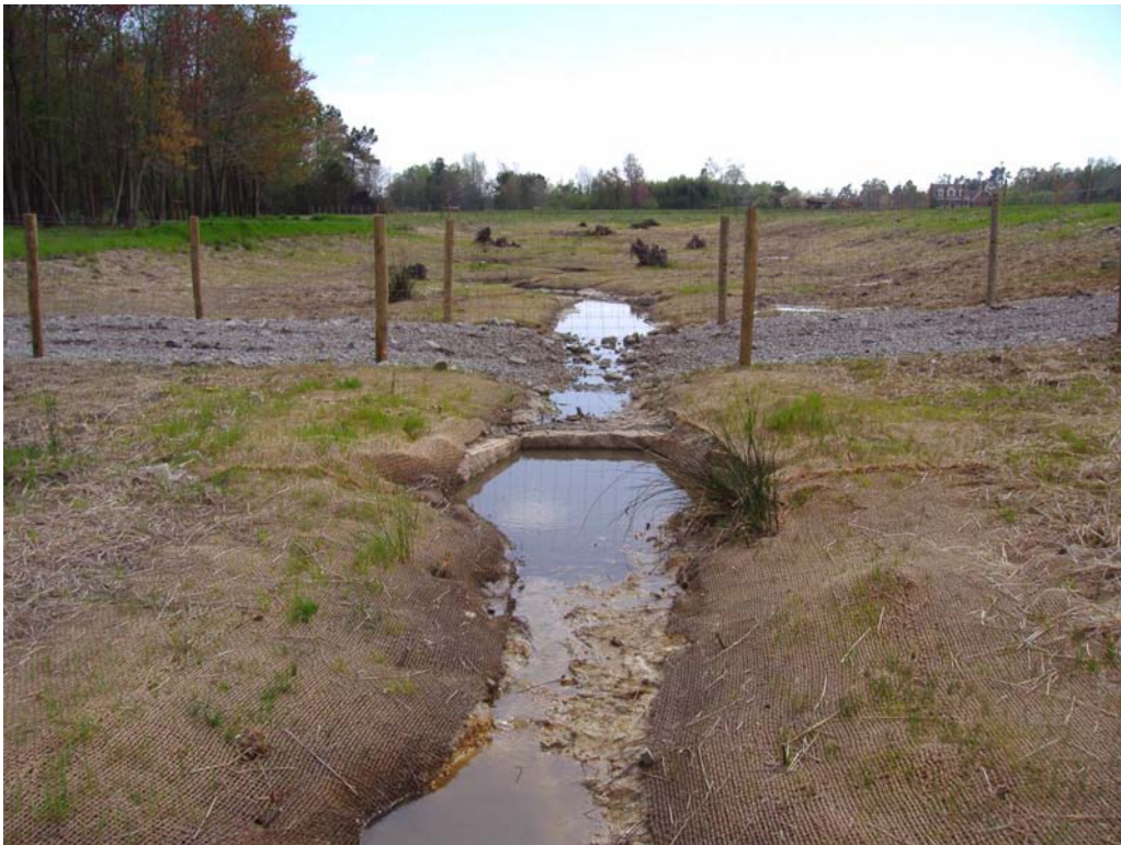
Photo Station 20. Ford Crossing – Upstream – Middle Reach
