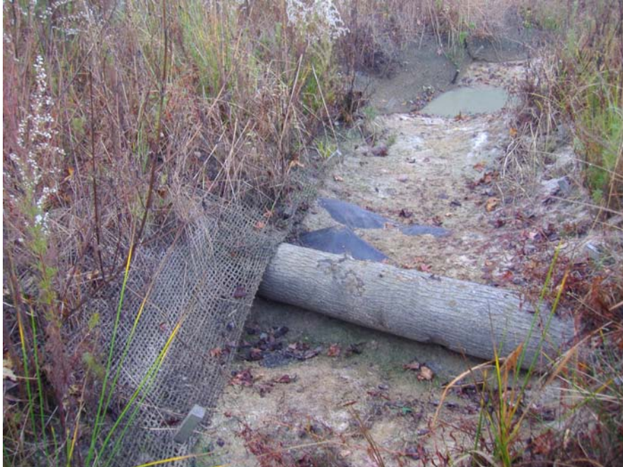
SP 3. Example of piping around a structure (STA 17+48)
