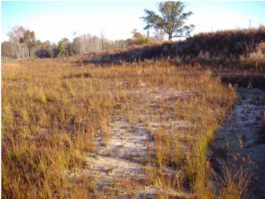
Photo VPA2: Bare area on floodplain near Middle Reach STA 20+30
