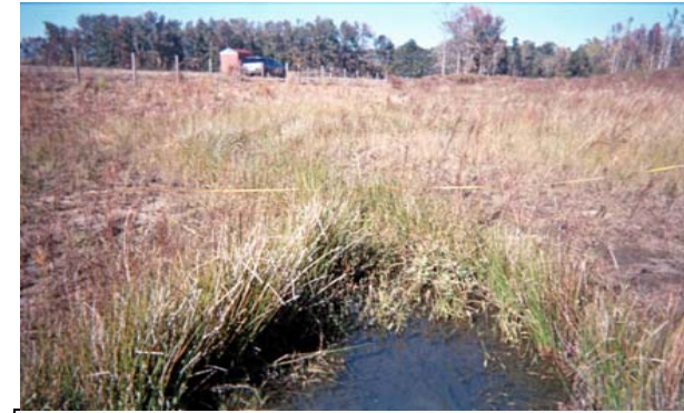
Photo of Cross-Section 5 - Looking Downstream @ STA 21+00
