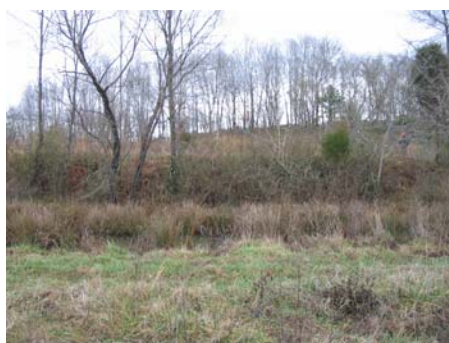
View of the old dam on UT2.
