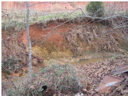
Bank erosion below the UT5 dam.
