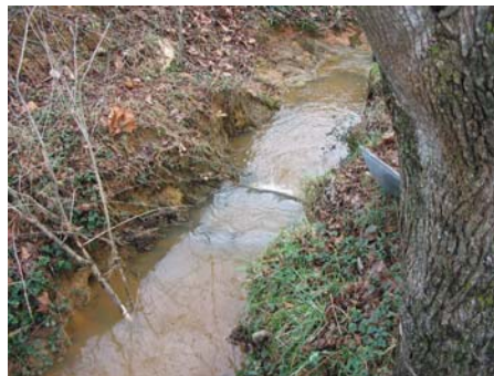
Headcut on UT5 below the old dam, view is downstream.
