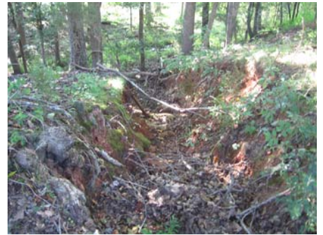
UT6 upper pond spillway, view is downstream.
