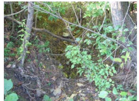
UT5 channel at the old dam below the proposed wetland creation.
