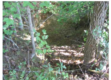
UT6 lower pond spillway above Mill Creek, view is downstream.
