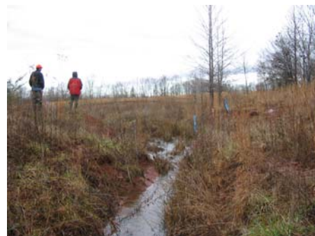
Outflow at the breached section of UT2, view is upstream.
