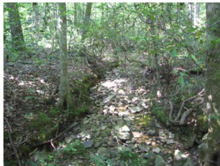
UT9 east of Lassier Mill Road culvert, view is downstream.
