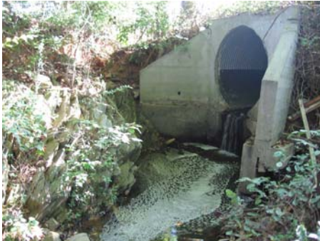
Beginning of the Mill Creek section at Lassiter Mill Road.
