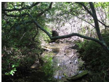
Mill Creek 3 at driveway culvert, view is upstream.
