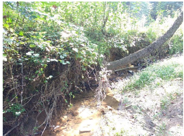
Photo 18: Undercut outer bank on UTHC3
