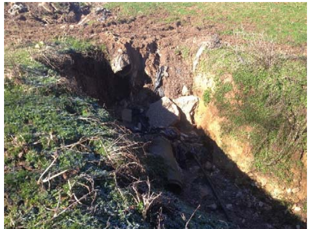
Photo 2: Beginning of T1 at culvert from pond
