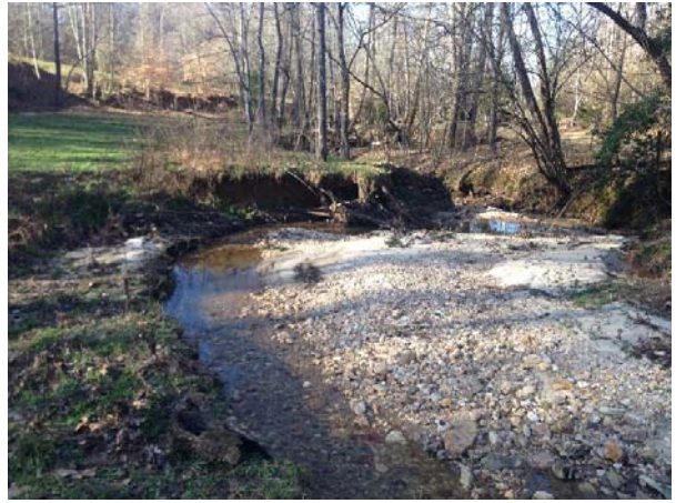
Photo 14: Active erosion and deposition on UTHC-3 downstream of confluence with T6
