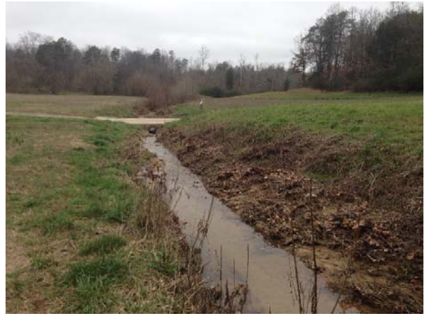
Photo 26. Downstream end of project on UTHC-4
