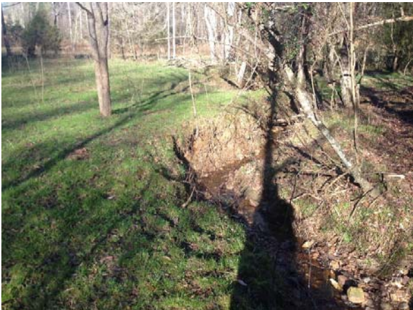
Photo 21: Entrenched portion of T7
