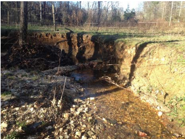
Photo 19: Active erosion on UTHC-3 just upstream of confluence with T7
