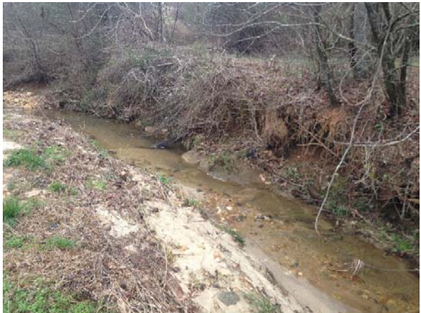
Photo 22: Active erosion on UTHC-4
