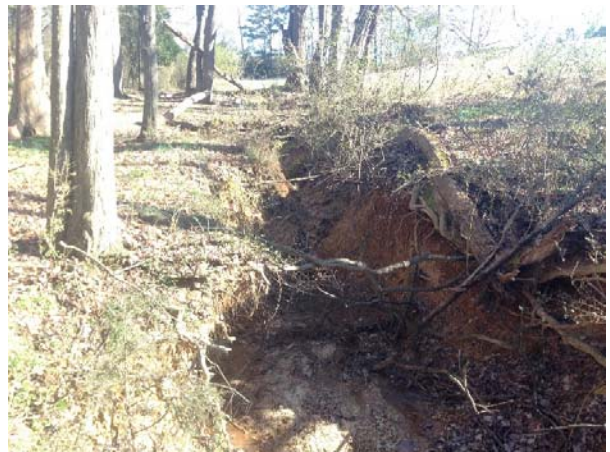
Photo 4: Headcut at beginning of T2
