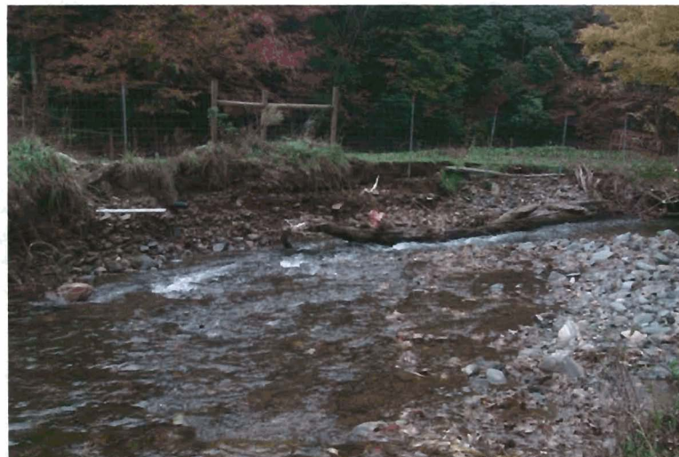
Bank damage after the series of hurricanes in September 2004.
