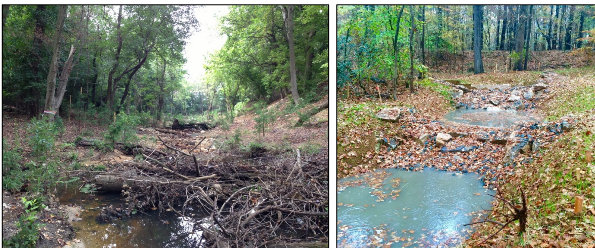
Figure 8.1: Step-Pool Systems with Underlying Sand Layer in Anne Arundel County, MD (left) and Durham, NC (right)
