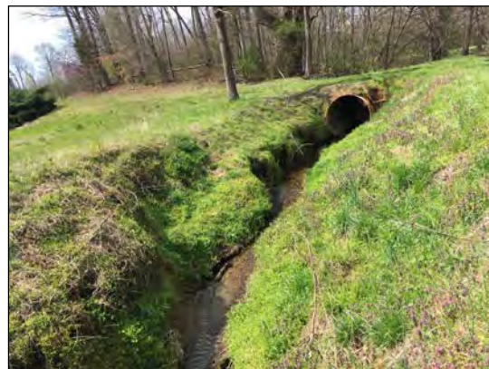
Culvert on Reach NM2 04/03/2018
