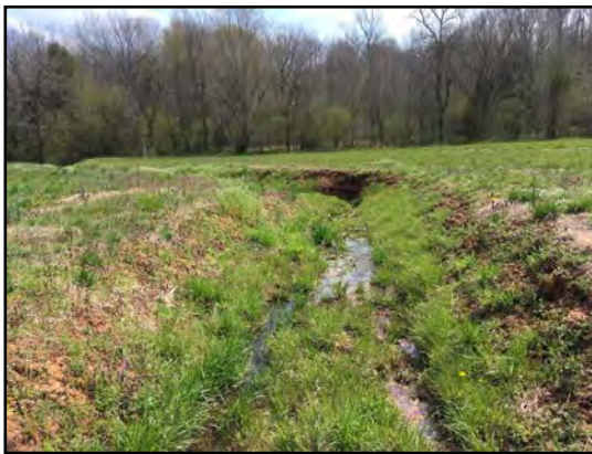
Looking downstream from culvert on NM3 04/03/2018
