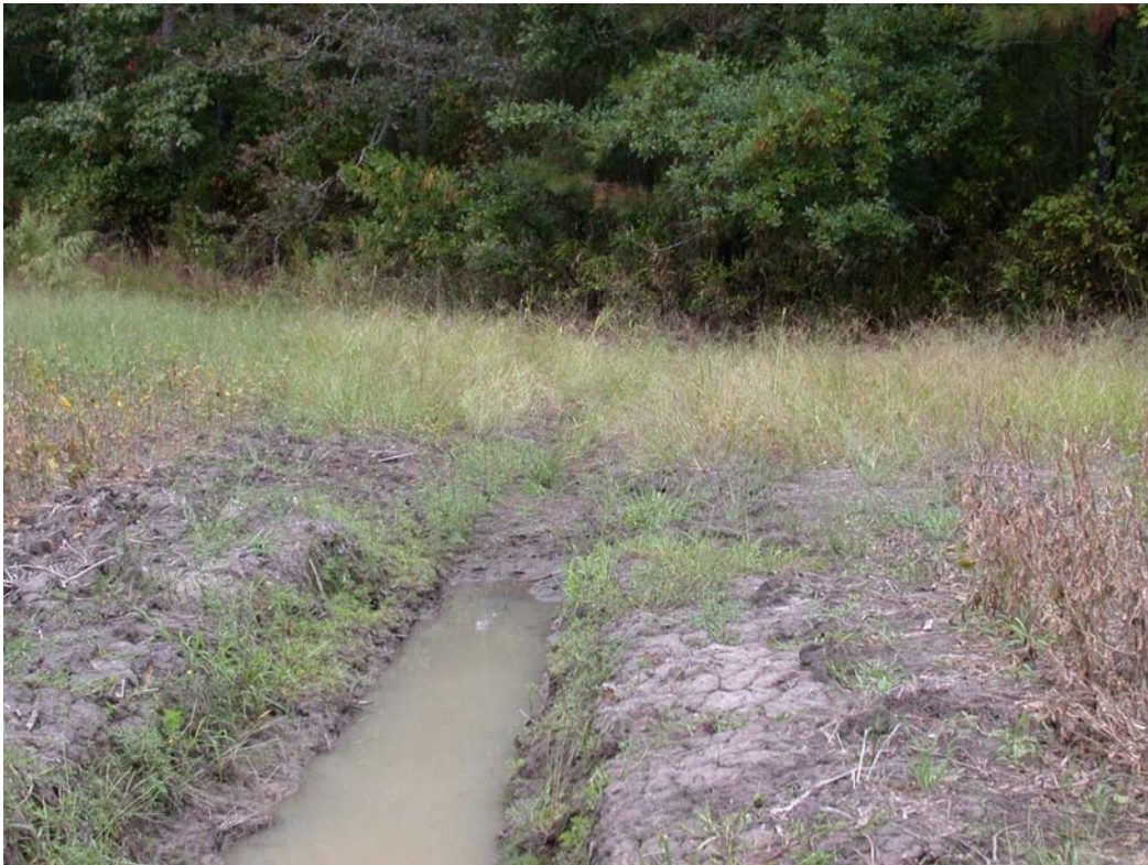
Photo 2. Upstream limits of ditch prior to construction.
