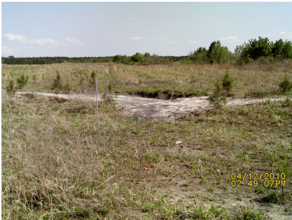
Reprofiling of berm near Gauge 1 to allow water onto site
