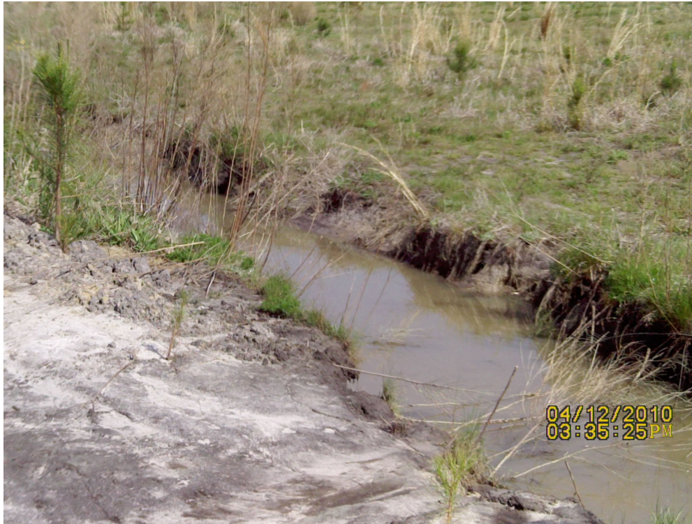
Ditch near Gauge 1 after plugging
