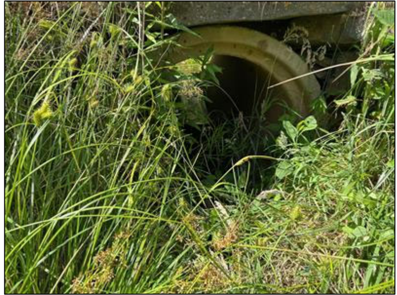
Culvert Looking Downstream
