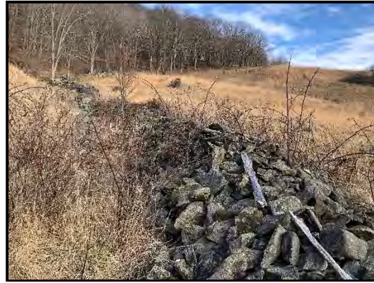
Reach G2 Looking upstream along the rock wall
