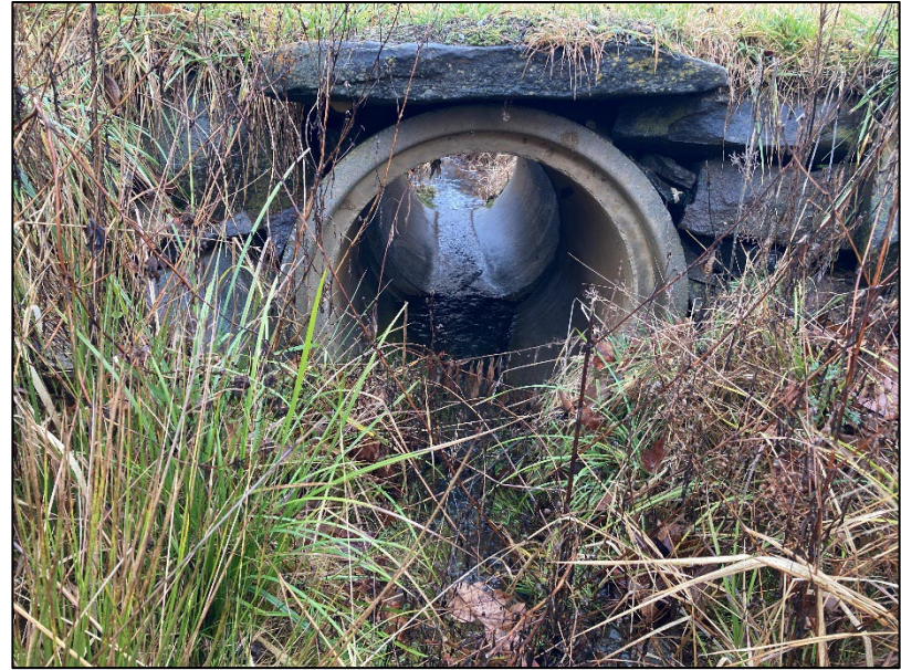
Culvert Looking Downstream
